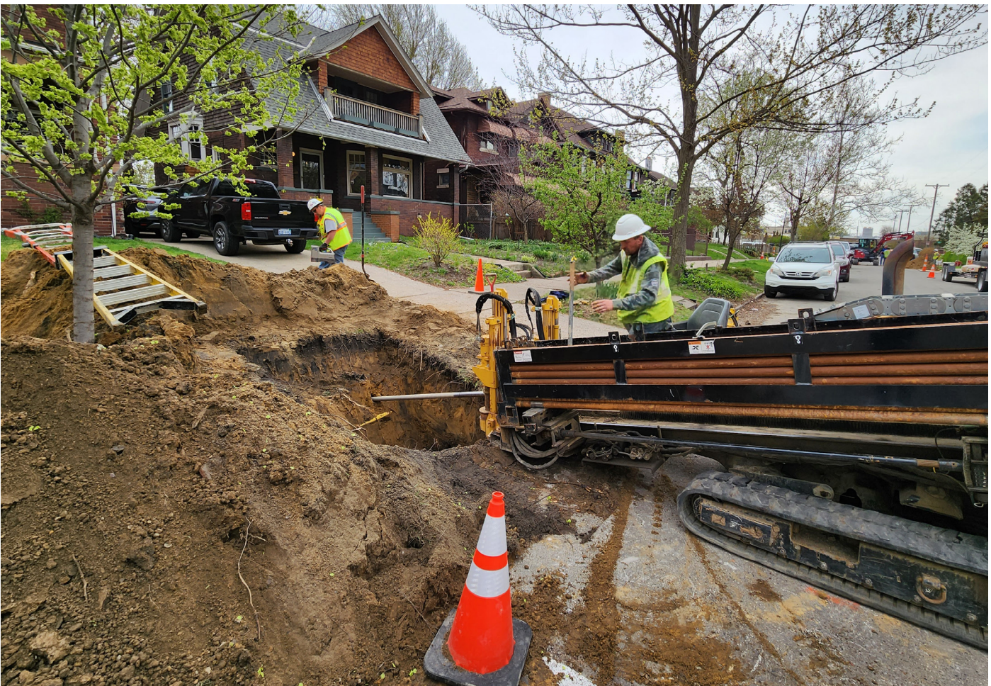
A DWSD contractor replaces a lead service line with copper.
