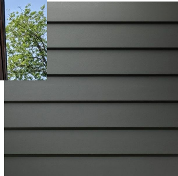
HARDI ARTISAN 6" LAP SIDING (SMOOTH) WITH MITERED CORNERS COLOR SHERWIN WILLIAMS NEEDLEPOINT NAVY SIDING
