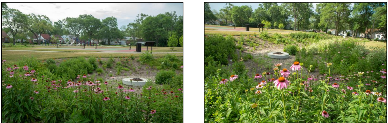
Figure 9 Liuzzo Park Bioretention Improvements
