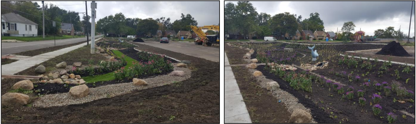
Figure 14 O'Shea Park Construction
