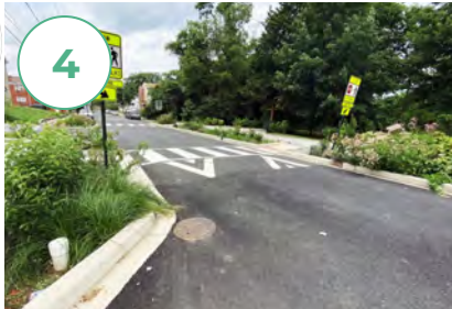
New Stormwater Connection
