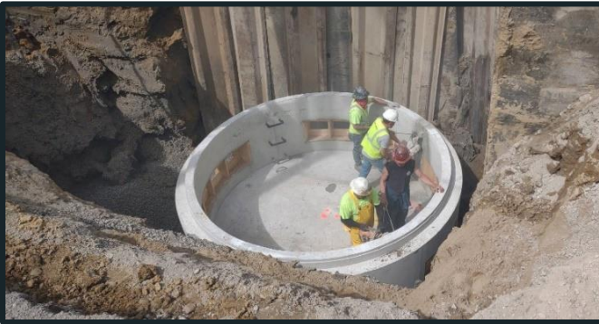
Storm sewer pipe installation on Sawyer Street.
