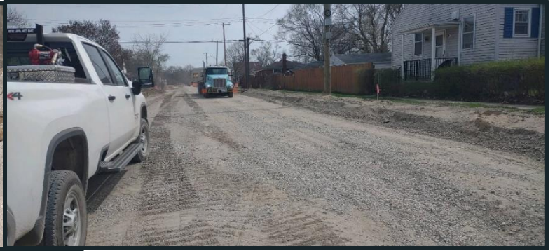
Road reconstruction work on the east end of Sawyer Street.
