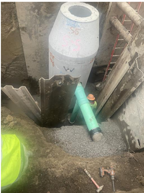
Combined sewer pipe and manholes being installed along Sawyer Street.
