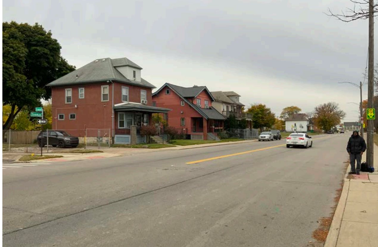
Room for improvement: Tireman Avenue is a mixed-use corridor that includes both businesses and housing, an active school and churches, and a bus line. But, its narrow sidewalks, wide roadway, and lack of street markings present safety challenges for walkers, bikers, bus riders, and drivers alike.
