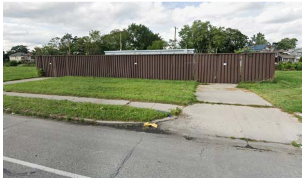
EXISTING PUBLIC LIGHTING SUBSTATION AT 6380 W. WARREN AVE.
