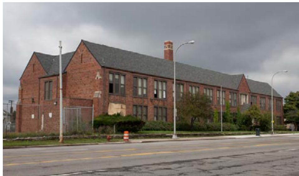
EXISTING RUTHRUFF SCHOOL BUILDING
