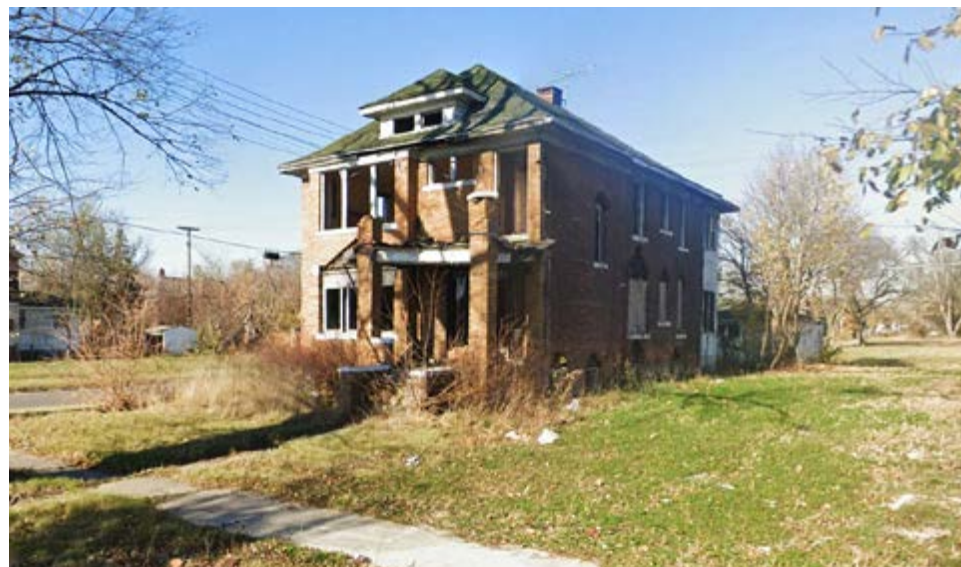
EXISTING VACANT SINGLE-FAMILY HOME AT 4686 PACIFIC AVE.
