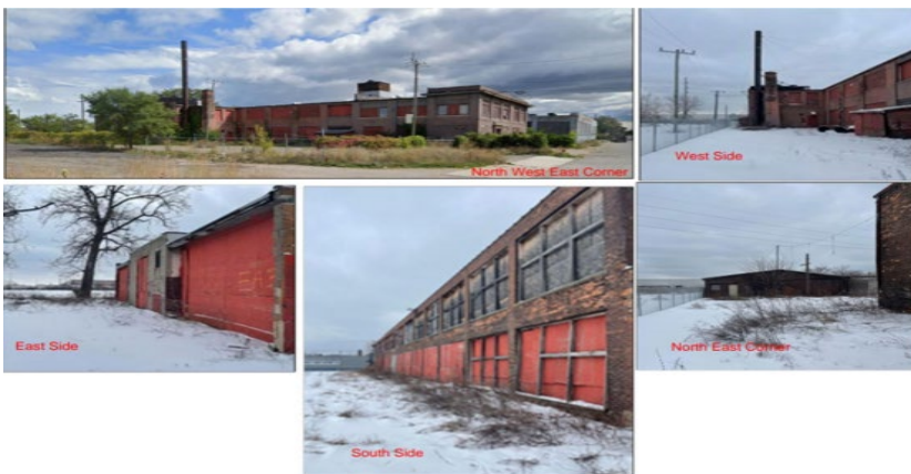
Figure 4 - Photos of 630 Lycaste Street, Detroit, MI 48214
