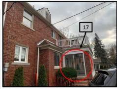
135 – Bedroom 2: Currently Single Hung without grid, putty color, seal broken causing condensation between panes Planned: Double Hung with grid, black color
