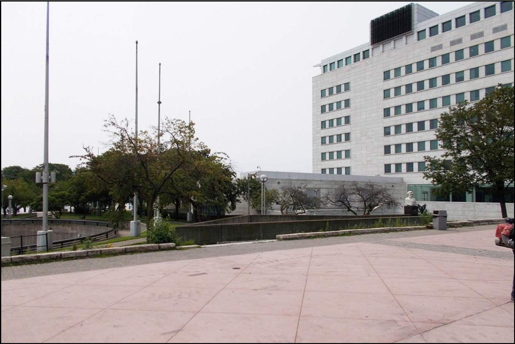
AT&T SITE UAW-FORD JOINT TRUSTS CENTER BUILDING LOCATION #1 (EXISTING)
