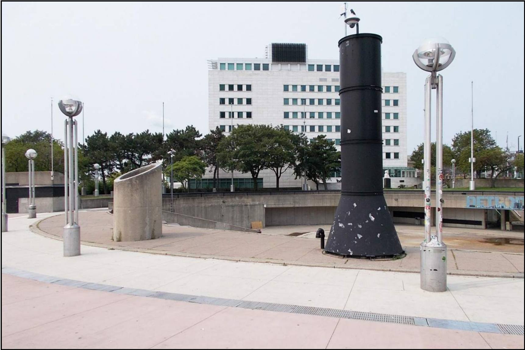
AT&T SITE UAW-FORD JOINT TRUSTS CENTER BUILDING LOCATION #2 (EXISTING)
