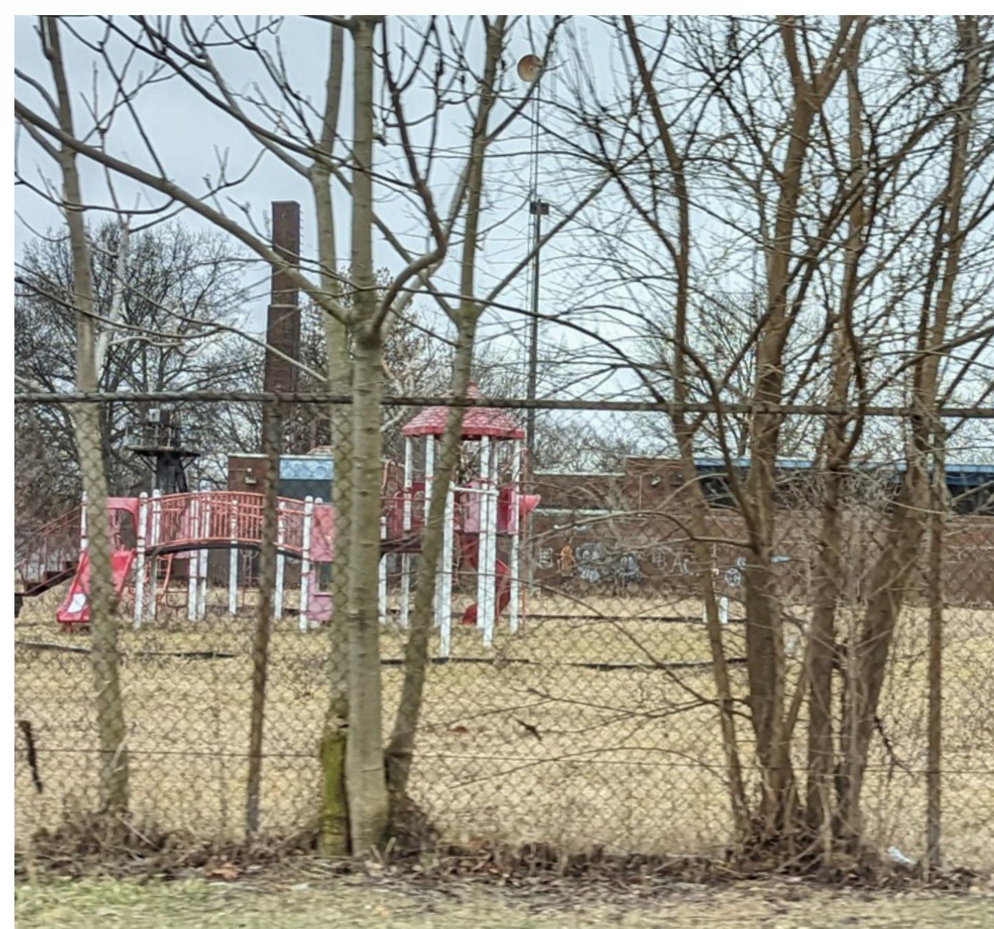
Vacant industrial buildings & industrial properties
