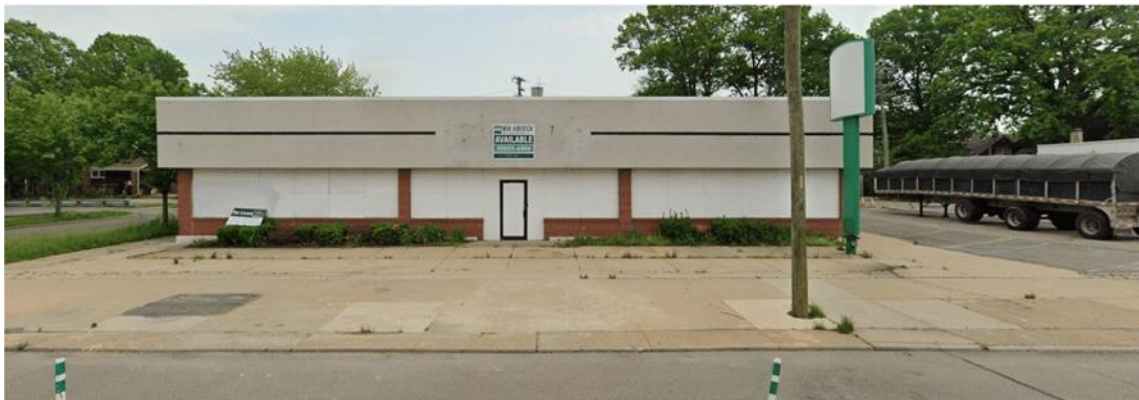
View of 16530 East Warren prior to demolition 15
