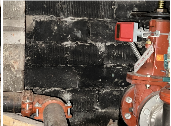
Figure 4. Foundation wall under entry stair.
