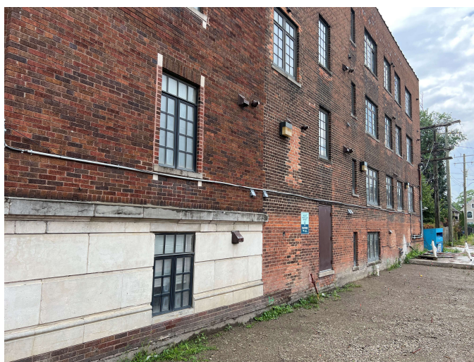
Figure 5. North wall along public alley.
