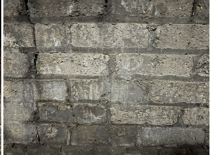
Figure 2. Foundation wall in lift shaft enclosure.
