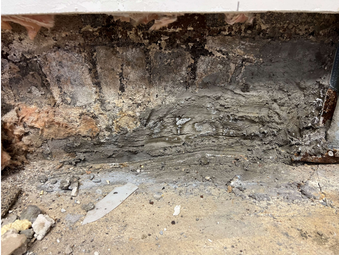
Figure 3. Foundation wall in laundry room.
