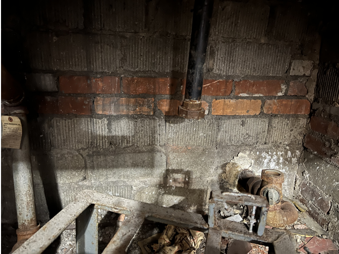
Figure 1. Foundation wall under North Stair
