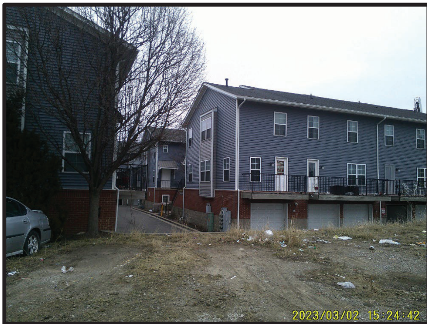
Photo 16. View of multi-tenant residential complex on the adjoining property to the east along Harper Avenue.
