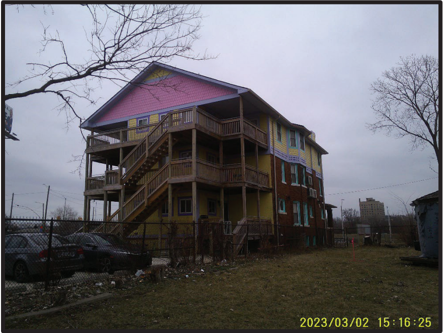
Photo 17. View of multi-tenet residential structure located on the east adjoining property along Edsel Ford Service Drive.
