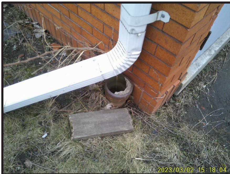
Photo 8. Stormwater drain for roof drainage at the unoccupied structure.
