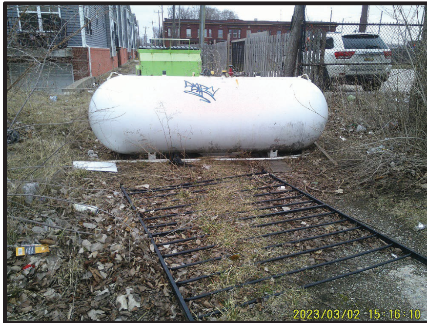
Photo 14. View of AST situated near the eastern edge of the Subject Property within the electrical utility easement.
