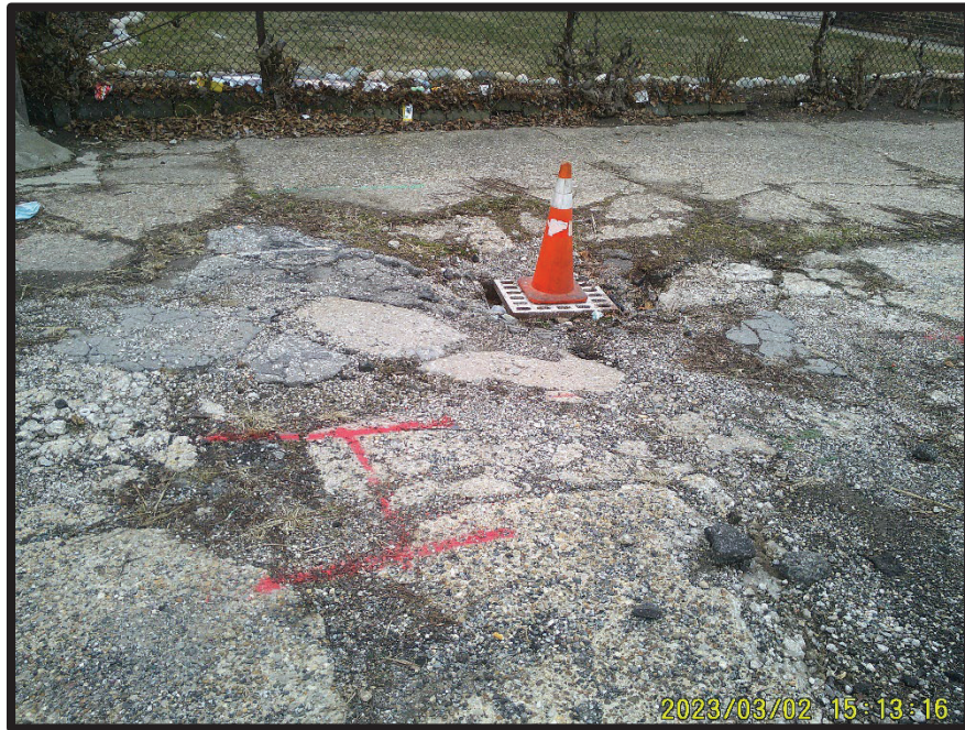
Photo 11. Typical view of stormwater drain located near the southeast corner of the Subject Property.
