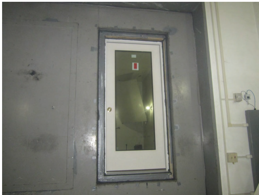
Source Room View of Installed Specimen
