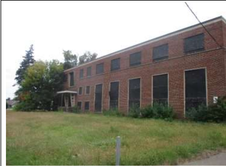
Photo 1. A view of the front of 17400 Meyers Road
