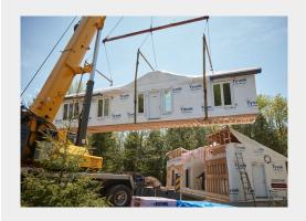
Bring down construction costs with 3D printing, manufactured or modular homes
