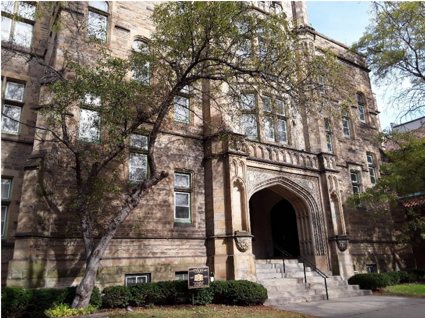
Southern exterior wall of the subject building
