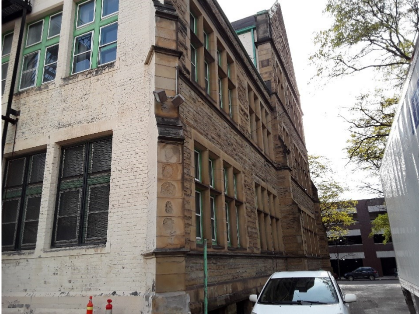
Western exterior wall of the subject building
