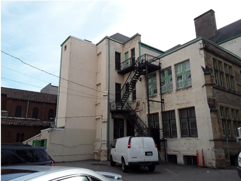
Northern exterior wall of the subject building
