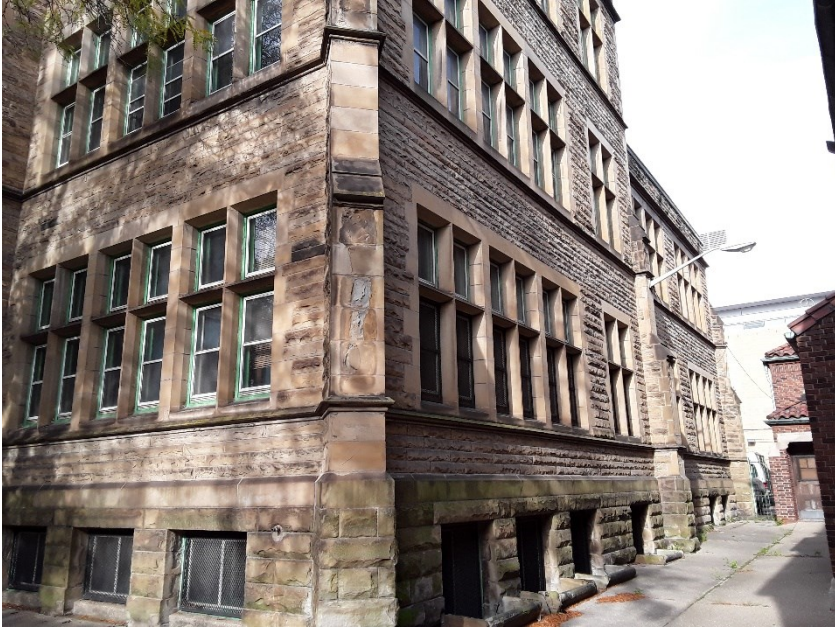
Eastern exterior wall of the subject building
