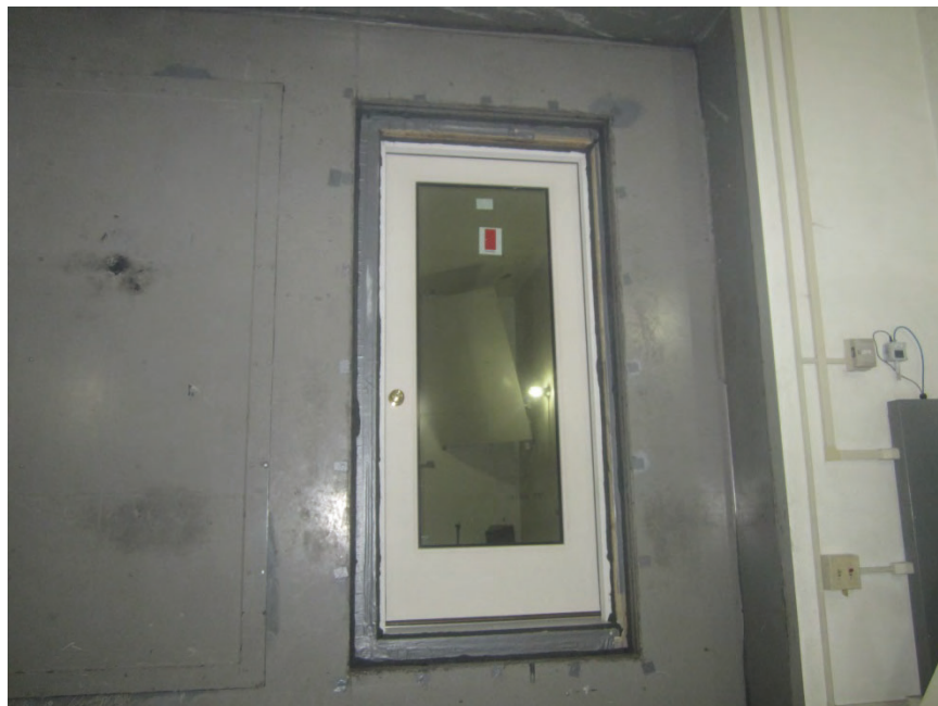
Source Room View of Installed Specimen
