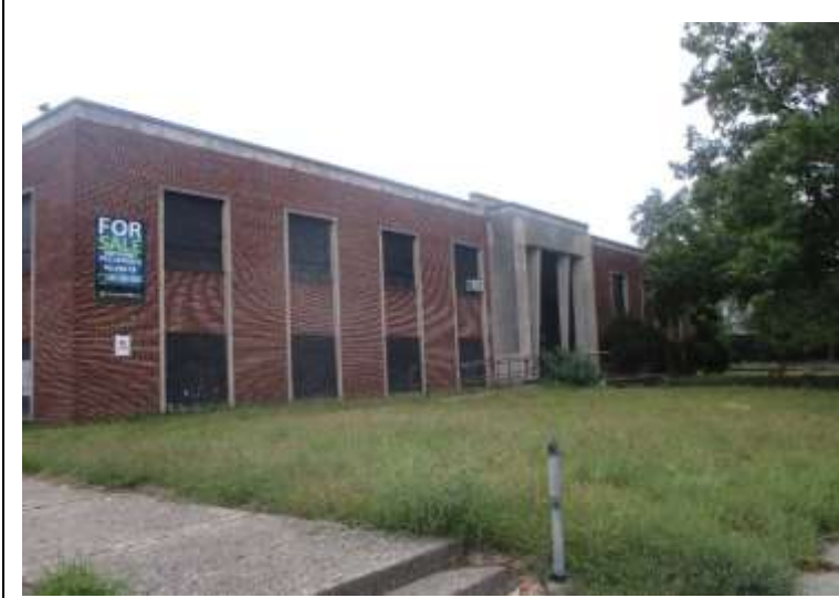
Photo 7. A view of the front of 17370 Meyers Road
