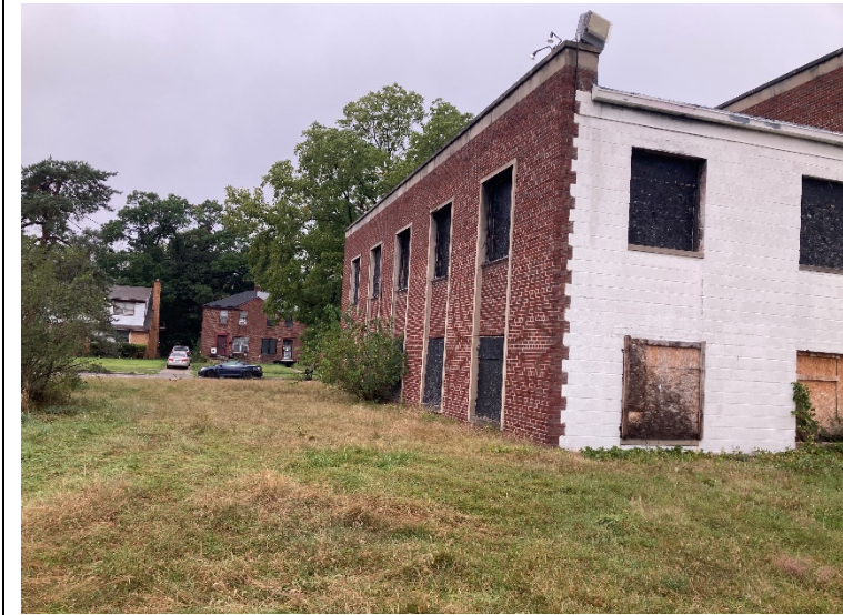
Photo 4. View of the side D of 17370 Meyer building.
