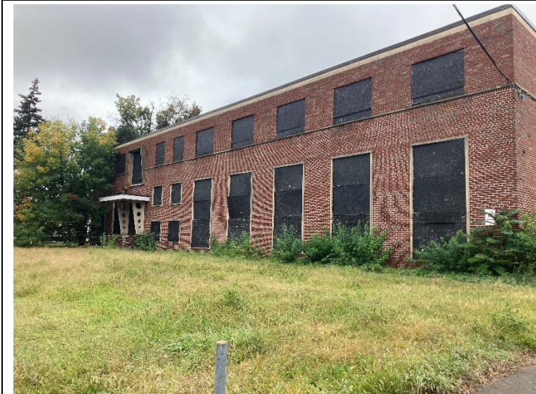
Photo 5. View of the side A of 17400 Meyer building.
