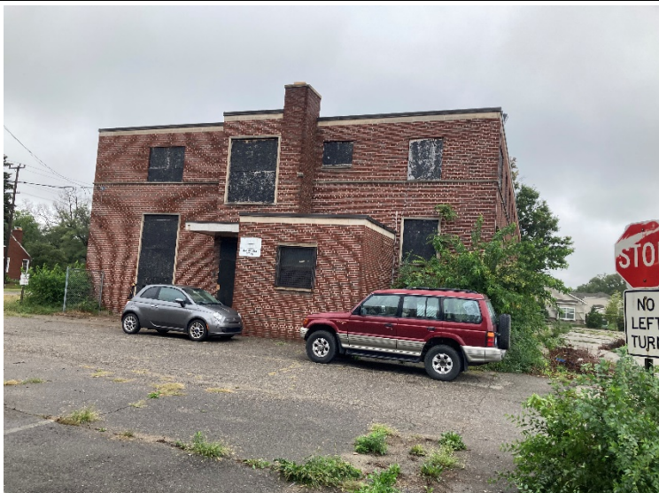
Photo 8. View of the side D of 17400 Meyer building.
