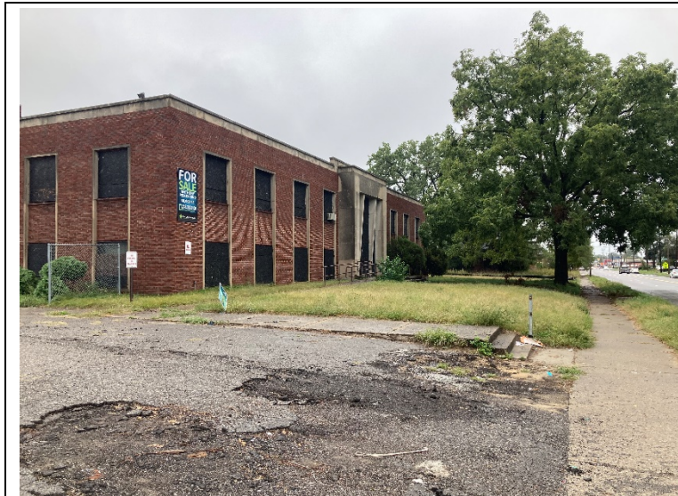
Photo 1. View of the side A of 17370 Meyer building.
