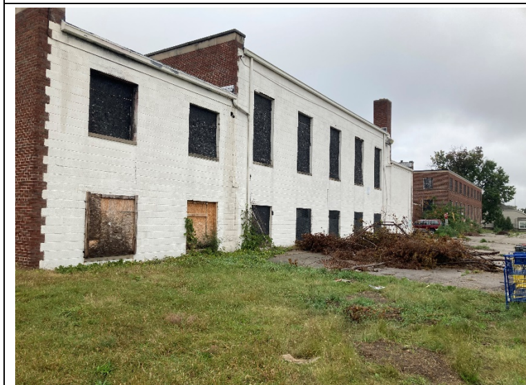
Photo 3. View of the side C of 17370 Meyer building.
