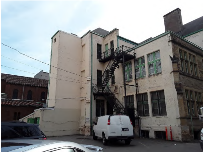
Northern exterior wall of the subject building
