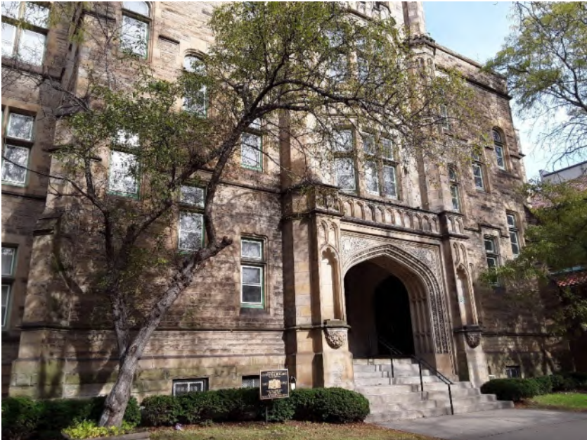
Southern exterior wall of the subject building
