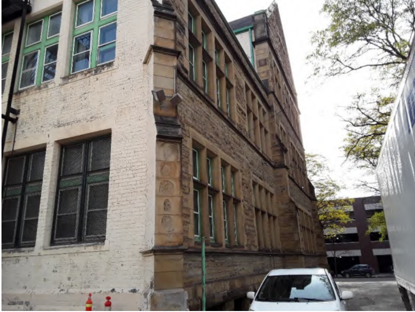
Western exterior wall of the subject building
