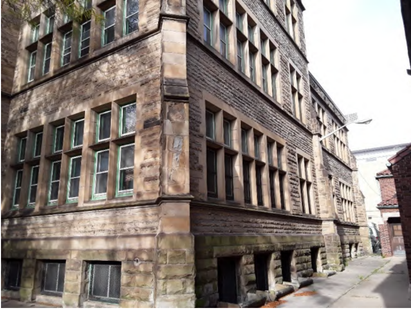
Eastern exterior wall of the subject building
