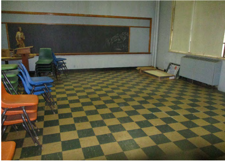
Photo 22. A view of asbestos-containing 9"x9" floor tile in room 102
