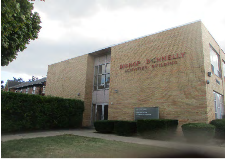
Photo 1. A view of the front of 5959 Whittier, Detroit
