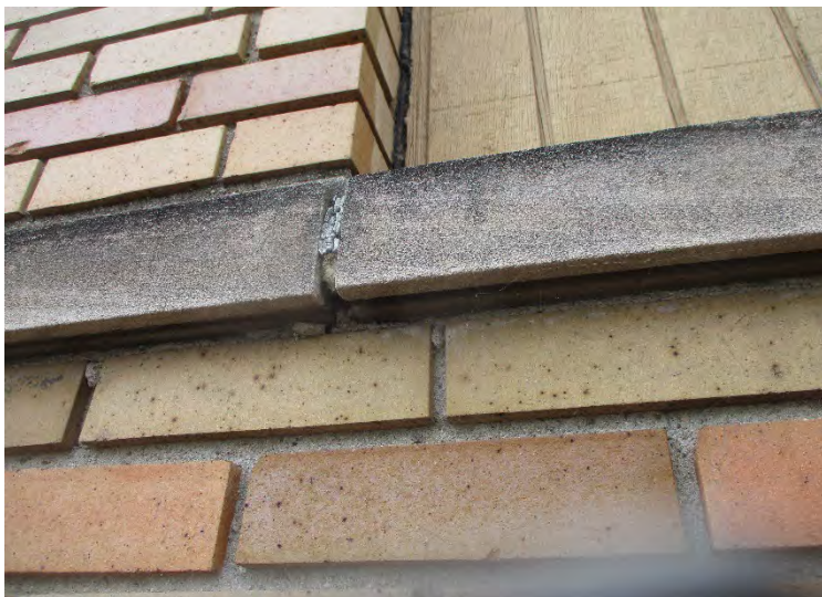
Photo 36. A view of asbestos-containing stone mortar
