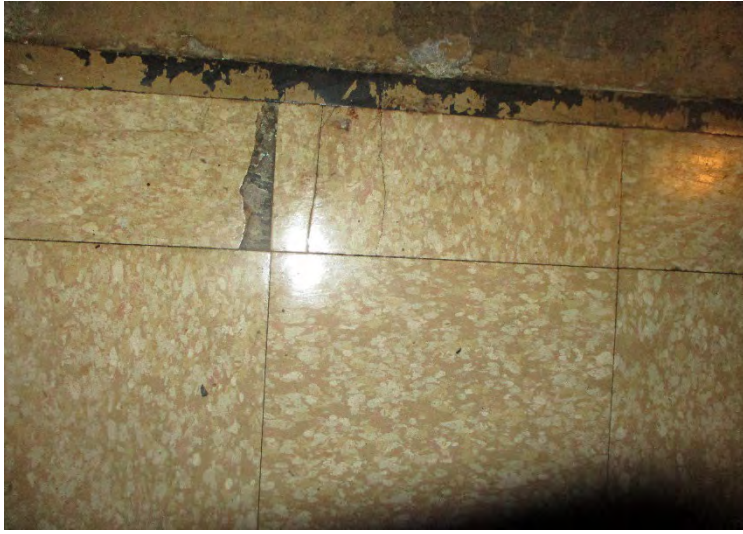
Photo 25. A view of asbestos-containing 9"x9" floor tile in room 104
