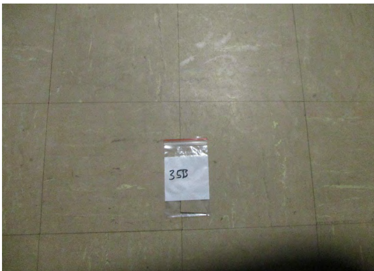
Photo 24. A view of asbestos-containing 9"x9" floor tile in room 112
