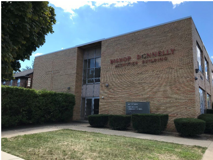
Photo 5. View the of the A side of the Activities Building on Whittier
