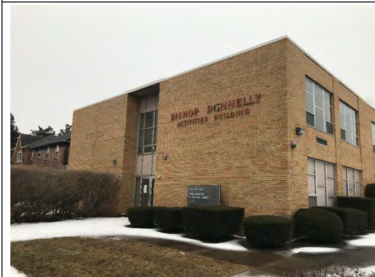
Photo 2. East side of School on Whittier
