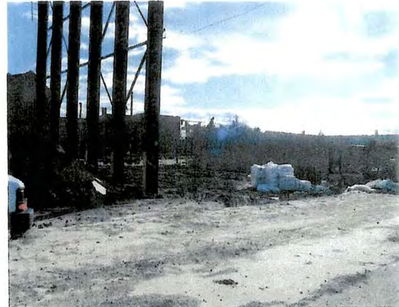
Vacant central part of property and new construction
