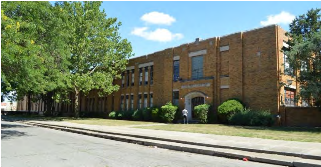
Photo 4 Looking northeast at front of school building, August 2022
