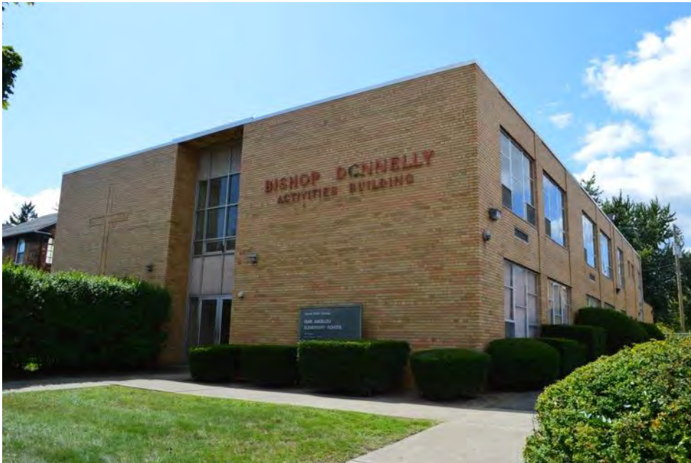
Photo 6 Looking southwest at Activities Building, September 2020
