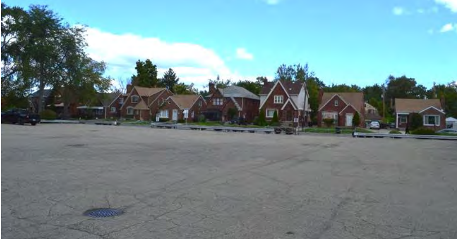
Photo 3 Looking east at existing parking lot, gates to be replaced, Chandler Park HD in background, September 2020
