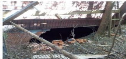
3184 Eastlawn STA b foundation 5-10-23.JPG
