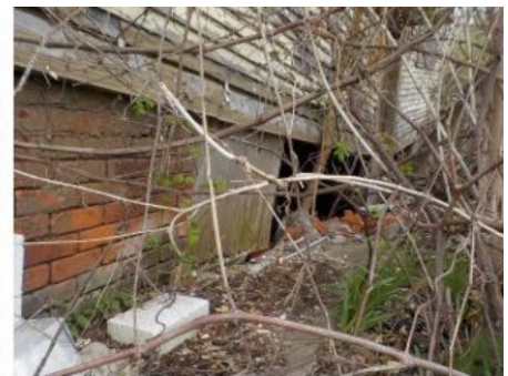
9337 Jameson STA b foundation 4-18-23.JPG
