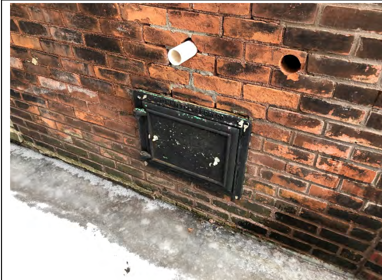
Photo 8. A coal chute identified on an adjoining dwelling
