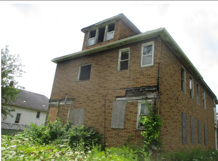
Photo 2. View of the 2544 – 2548 Van Dyke Street rear
