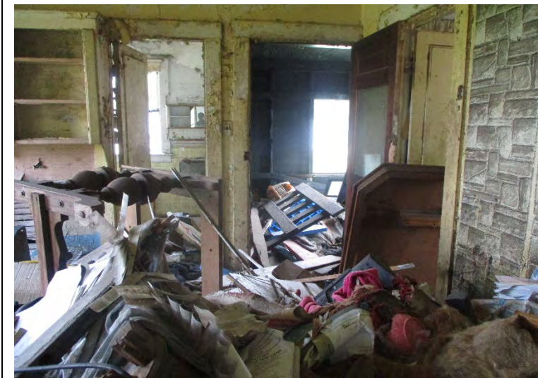
Photo 5. View of interior
