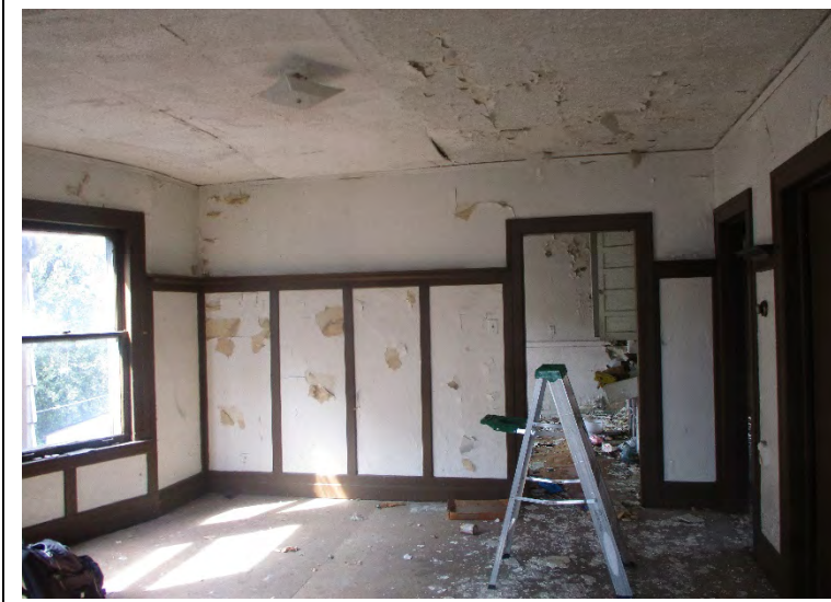
Photo 4. View of the 2463 – 2465 Seyburn Street interior
