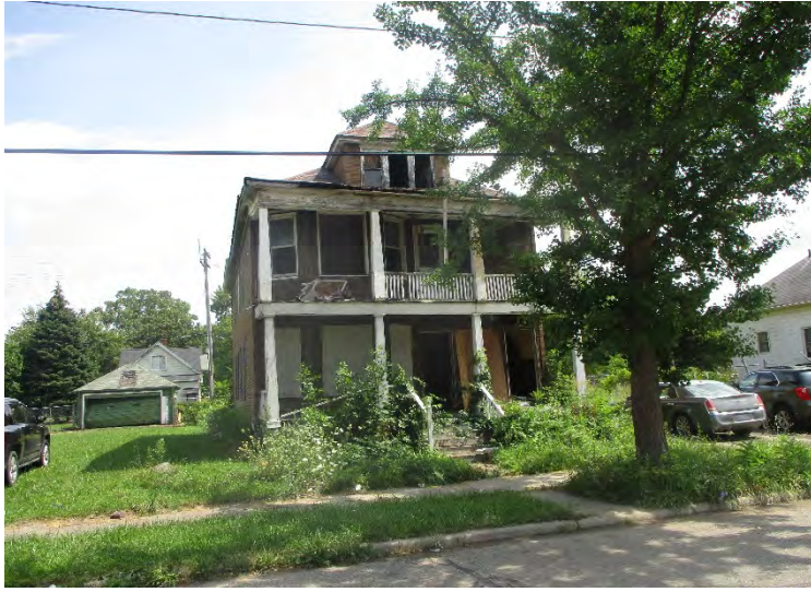
Photo 1. View of the 2544 – 2548 Van Dyke Street front
