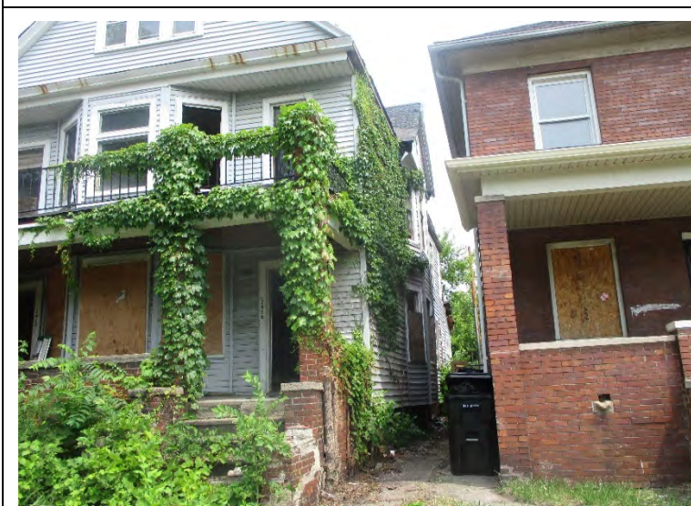
Photo 2. View of the 2406 – 2410 Baldwin Street south side
