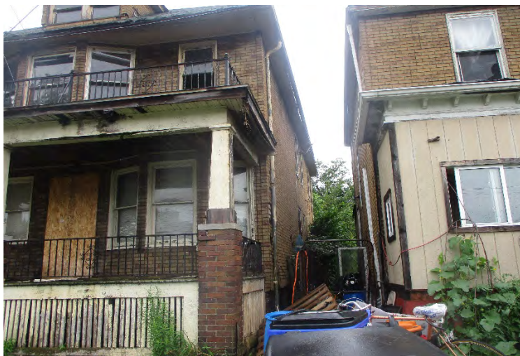
Photo 3. View of the 2463 – 2465 Seyburn Street north side
