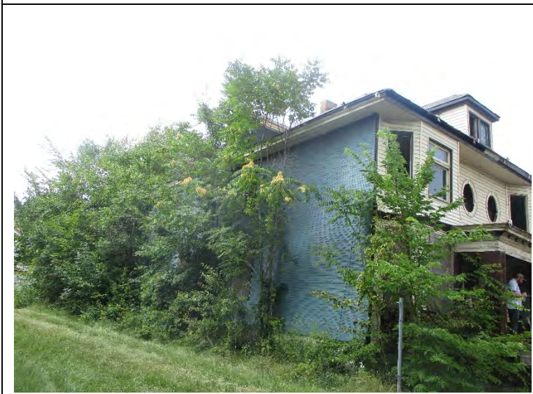
Photo 2. View of 2251-2253 Sheridan Street south side
