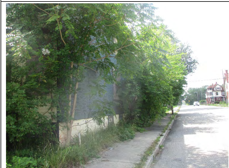
Photo 3. View of 2251-2253 Sheridan Street north side
