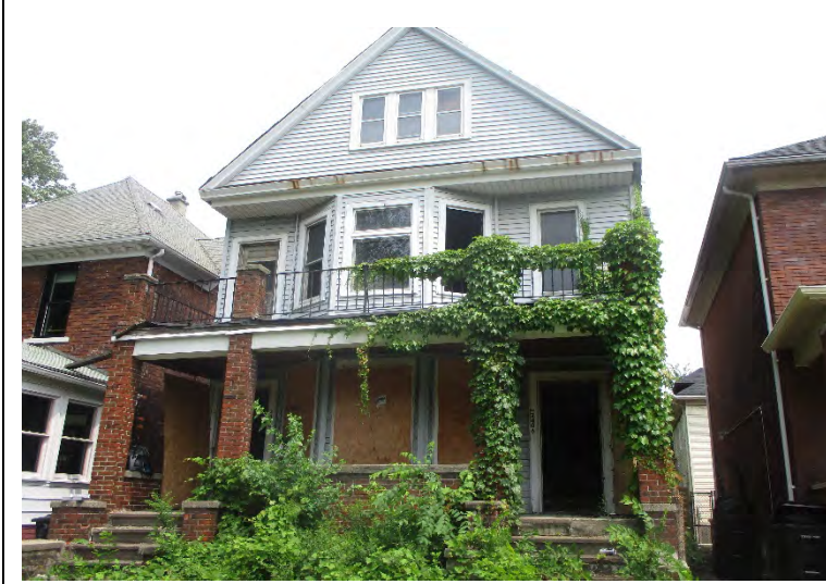
Photo 1. View of the 2406 – 2410 Baldwin Street front
