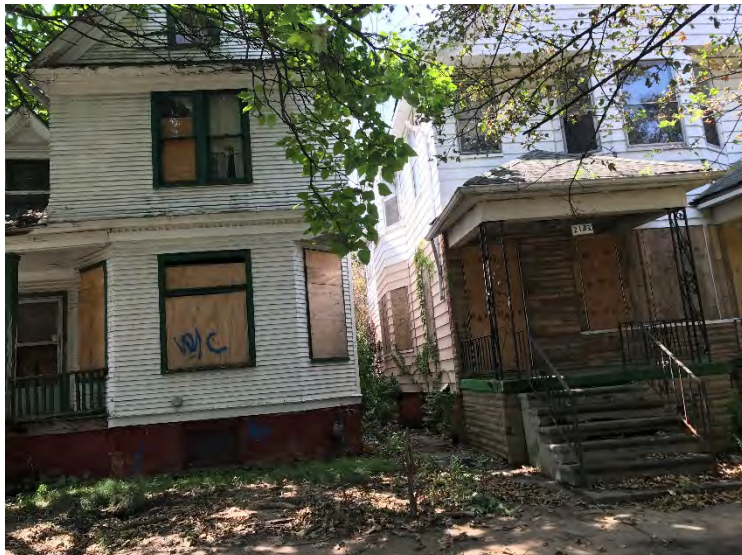
Photo 2. View of 2143-2145 Townsend south side
