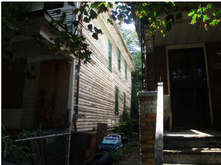
Photo 3. View of 2419-2423 Beals Street north side
