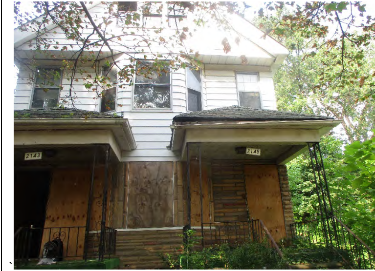
Photo 1. View of 2143-2145 Townsend front
