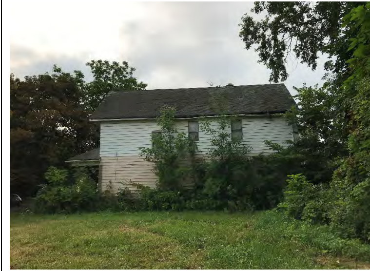
Photo 4. View of 2143-2145 Townsend north side.
