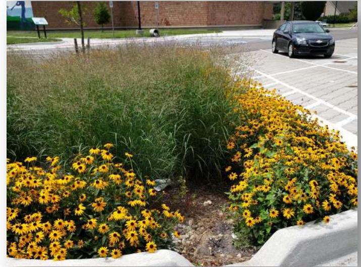
Porous pavers and bioswales within Crowell Recreation Center's parking lot
