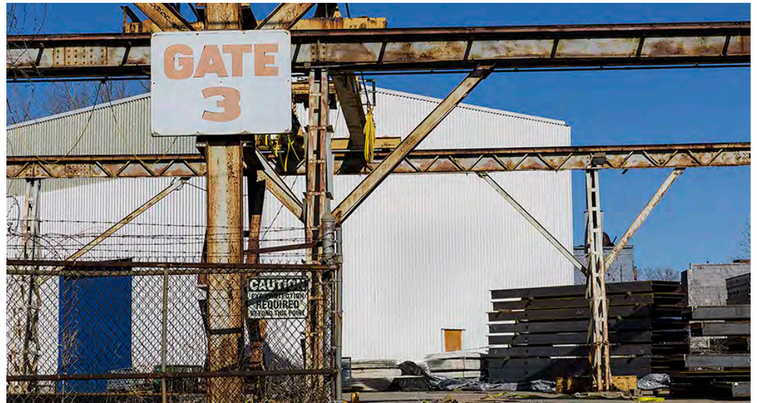
Industrial spaces in the Jeffries-Southfield Industrial District
