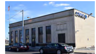
Central Savings Bank (1926) 18203 Fenkell
