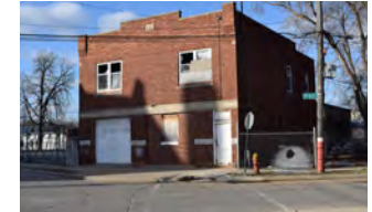
Former Fire Station & Redford Village Hall (1921) 22050 Argus
