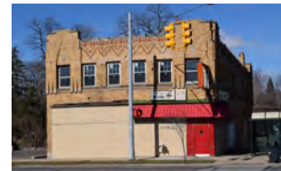
Occupied Building (1930) 18200 Grand River
