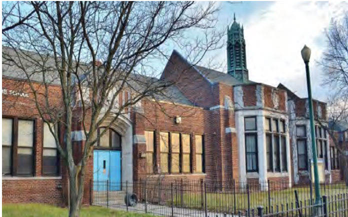
Former Holcomb Elementary School in 2017
