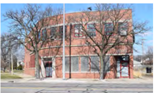
Occupied Building (1949) 15732 Grand River
