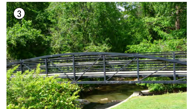
Bridges (Photo by Daniel Mayer, 2011)
