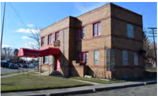
Occupied Building (1939) 20526 Grand River
