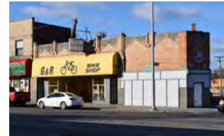
Occupied Building (1931) 21702 Grand River
