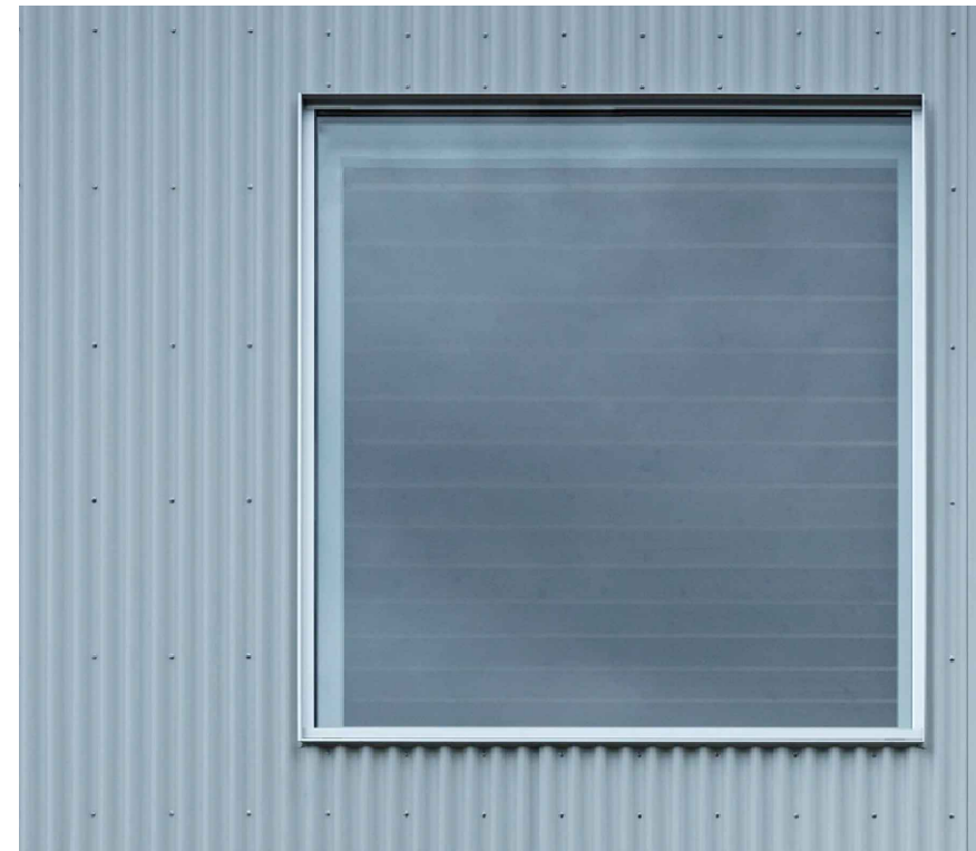
Corrugated Metal Panel / Window
