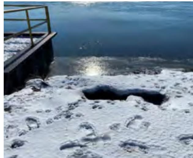
Unformed concrete poured along portions of shoreline is undermined
