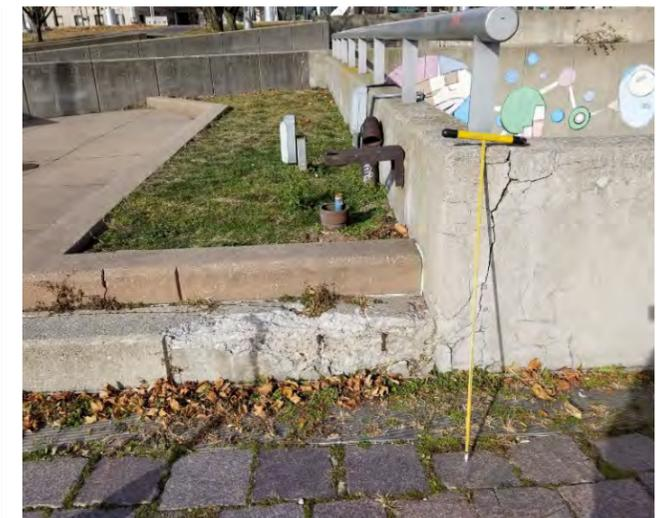
Fire and water damage to outside masonry wall in recessed area. Significant damage to painted surfaces
