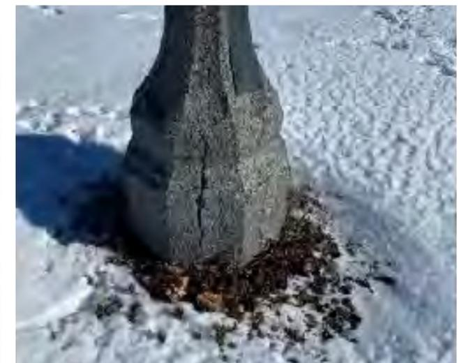
Precast concrete lighting fixtures with vertical cracking
