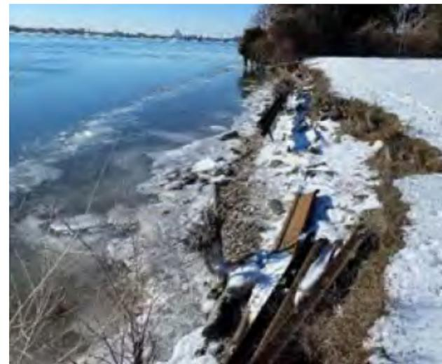
Guardrail section along shoreline is damaged and portions are missing, a potential hazard
