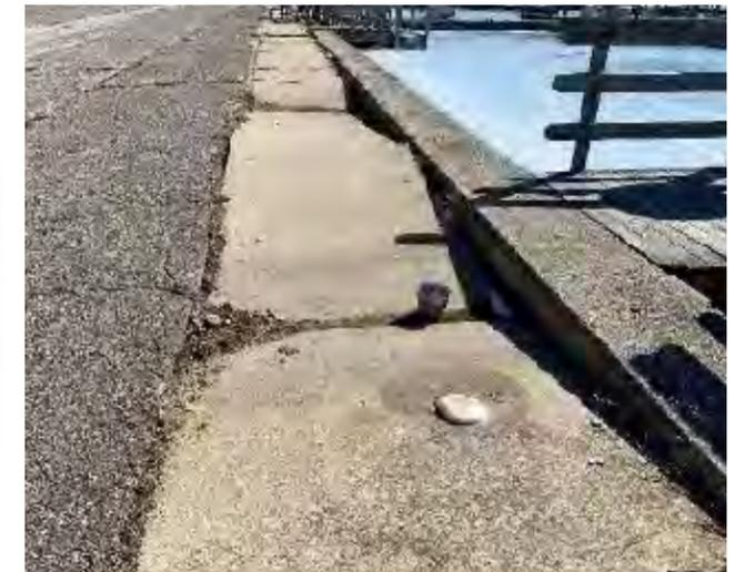
Significant settlement behind wall causing concrete walk to be uneven and potentially hazardous
