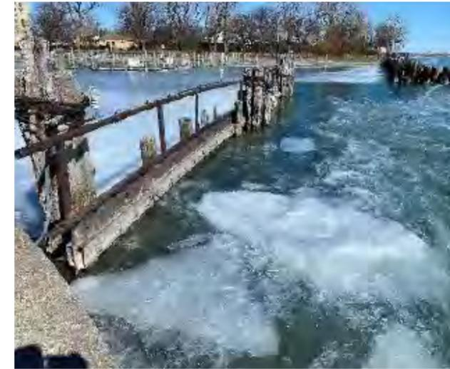
Timber pile and steel components noted to be in poor condition for breakwall at riverside entrance
