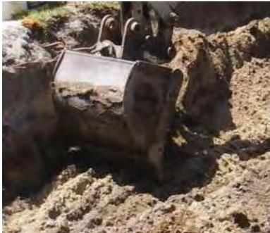
**Figure 8-37** Scarifying soil with a toothed excavator bucket
