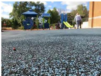
**Figure 10-9 Example Rubber Overlay**
