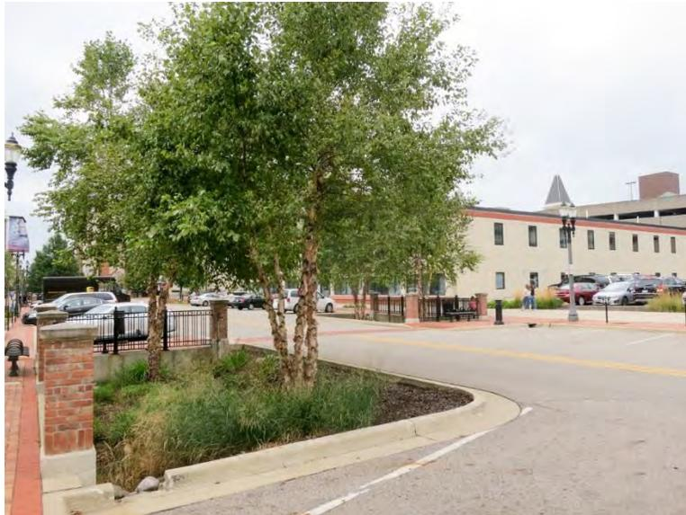
*Figure 15-9 Curb bump out bioretention with trees*
