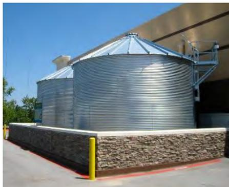
*Figure 3-4 Use of cisterns for water reuse*
