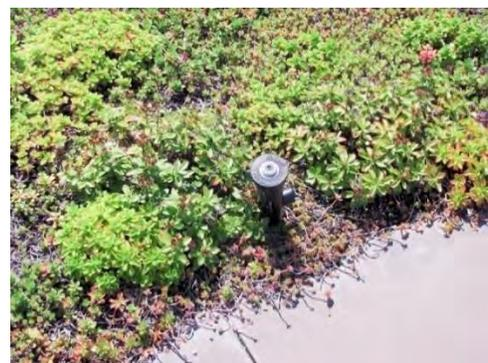
*Figure 12-21 Overhead spray irrigation on vegetated roof*
