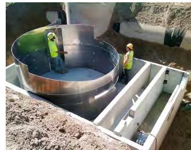
**Figure 9-13** Installation of typical manufactured treatment device
