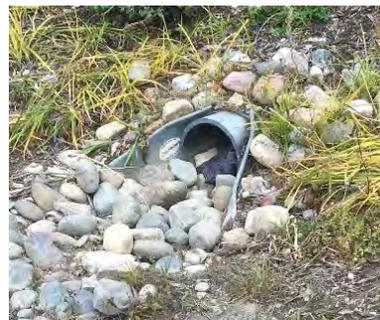
**Figure 8-22** Piped inlet
