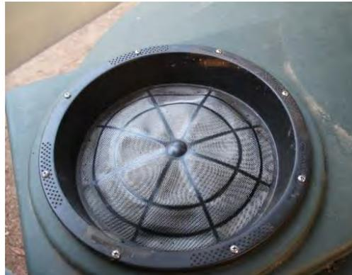
Figure 10-5 Filter at the Inlet on a Cistern
