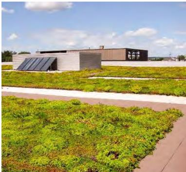
**Figure 12-22 Concrete paver paths for maintenance access**
