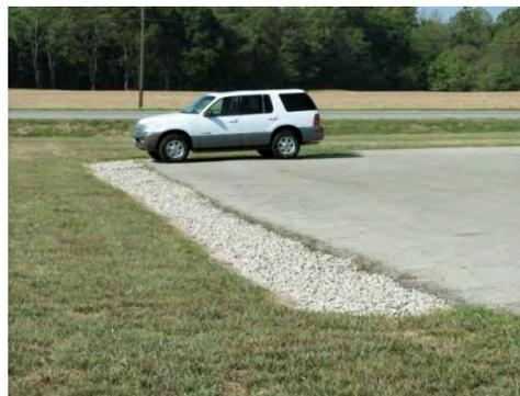
Figure 9-5 Infiltration Trench
