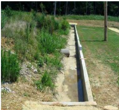
**Figure 9-10 Typical level spreader**
