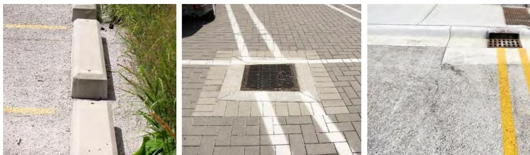
Pervious concrete parking; overflow conveyance to bioretention
