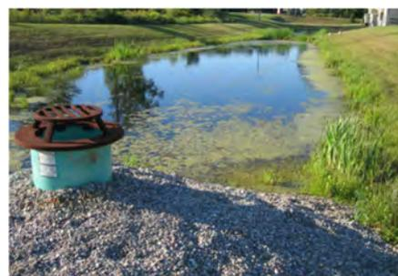
**Figure 1-3 Retention basin with outlet riser**
