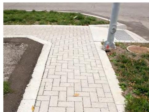
Figure 10-13 Permeable Sidewalk
