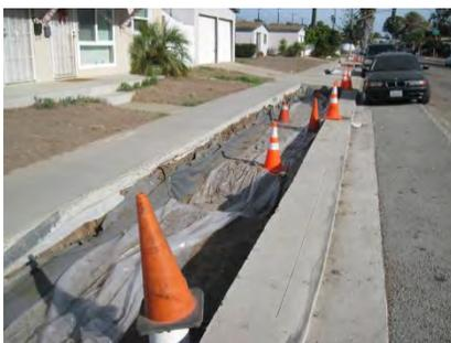
**Figure 10-34 Protection of subgrade during construction**
