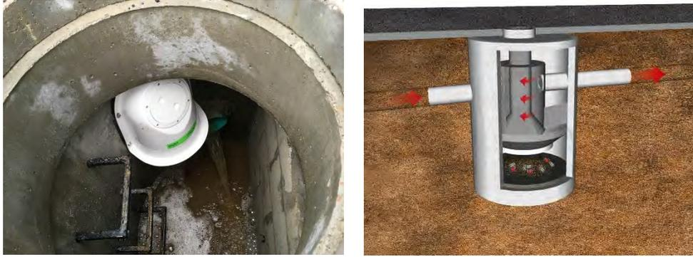
Figure 5-9 Gross Solids Removal Devices
