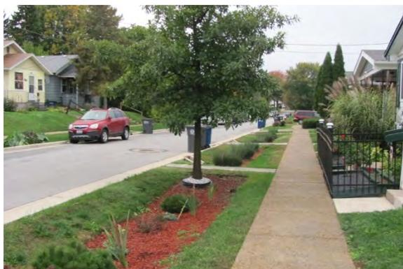
**Figure 8-9** *Linear Bioretention Along Roadway*
