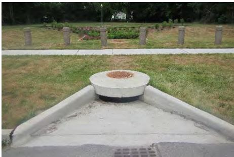
*Figure 8-19 Curb cut bypassing CB*
