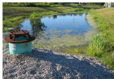
**Figure 1-3 Retention basin with outlet riser**
