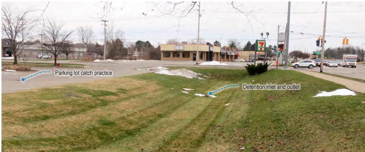
**Figure 7-4 Example detention practice with inlet and outlet as the same structure**
