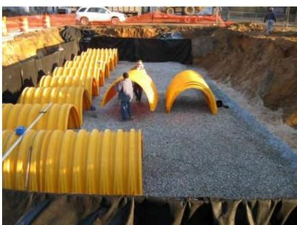
**Figure 9-4 Infiltration Vault**
