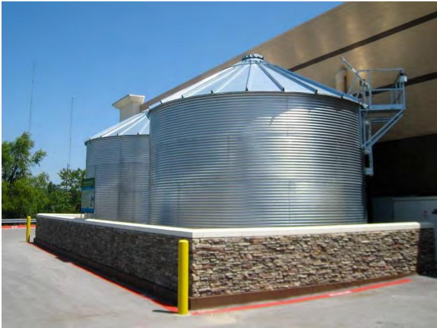
*Figure 11-1 Cistern Example Used for Irrigation*
