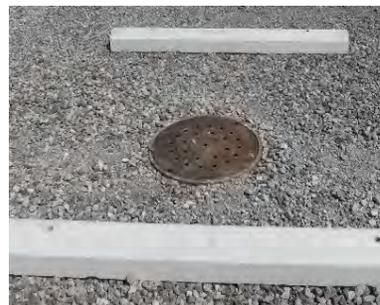
*Figure 8-26 Permeable aggregate parking lot outlet structure*
