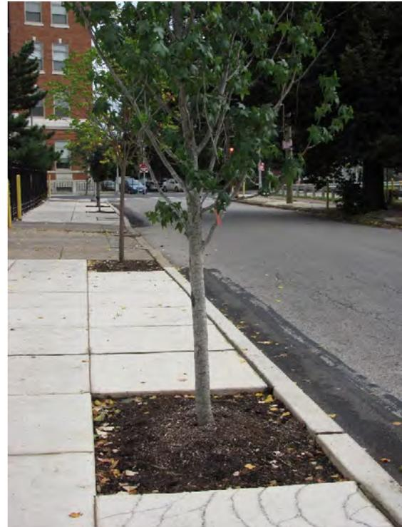
*Figure 8-6 Suspended Pavement Sidewalk*
