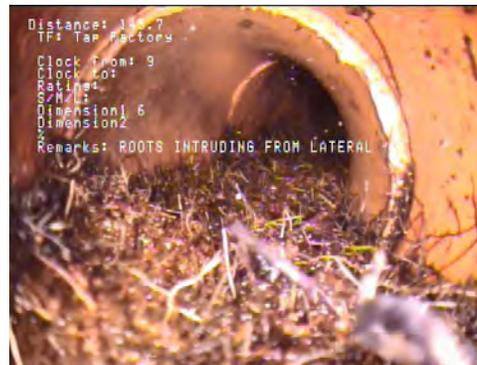
**Figure 15-15 Example root growth in sewer**
