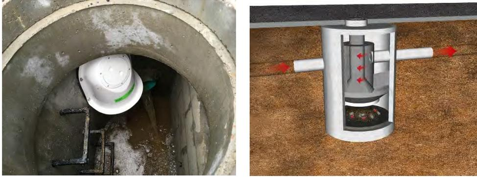
Figure 5-9 Gross Solids Removal Devices
