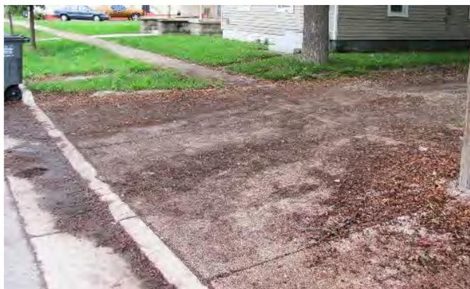
**Figure 10-16 Permeable pavement with significant leaf litter**
