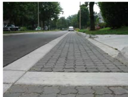
*Figure 1-5 Permeable concrete pavers*
