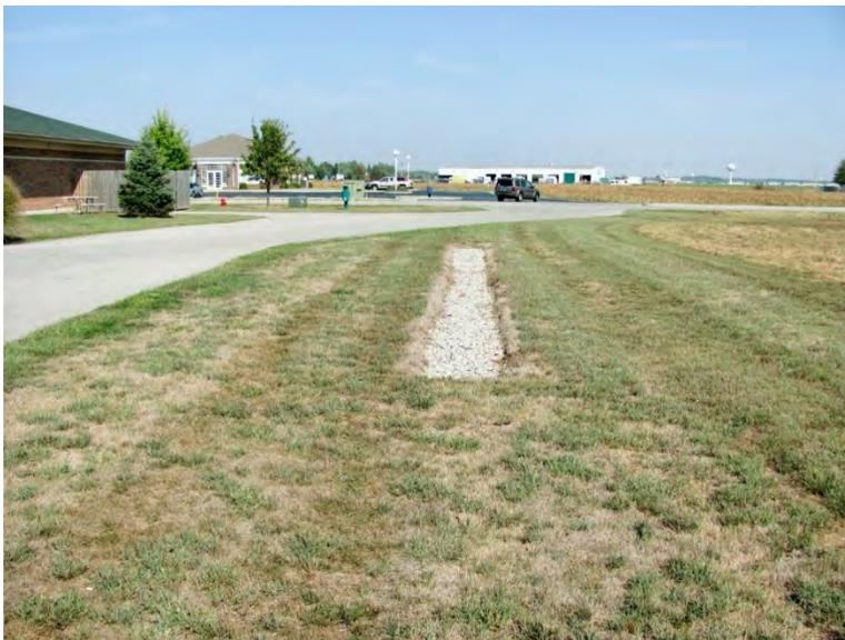
*Figure 9-1 Infiltration trench installed adjacent to drive lane*
