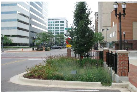
**Figure 8-10 CBD Curb Extension Bioretention**
