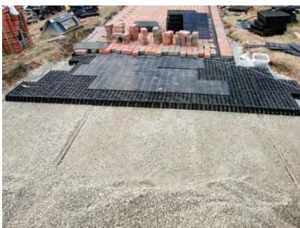
Figure 9-3 Infiltration Bed
