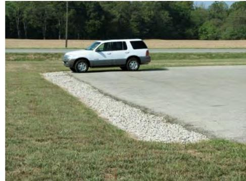
Figure 9-5 Infiltration Trench
