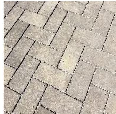
**Figure 10-5 Example of Permeable Interlocking Concrete Pavers**
