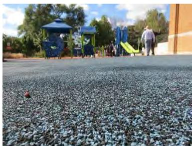
**Figure 10-9 Example Rubber Overlay**
