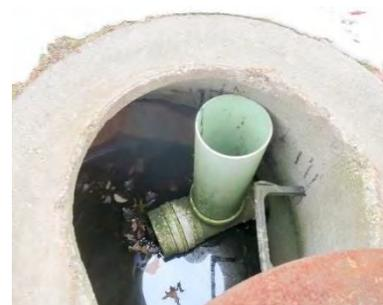
**Figure 10-26 Upturned underdrain with a capped tee connection**
