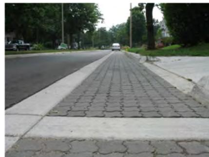
*Figure 1-5 Permeable concrete pavers*
