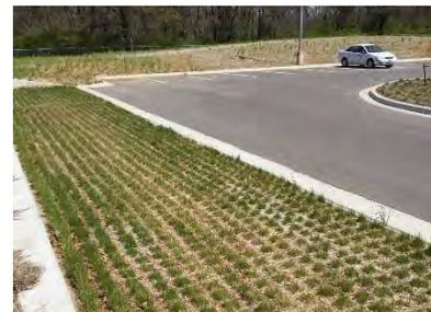
**Figure 10-6 Example of Grid Pavement Systems**
