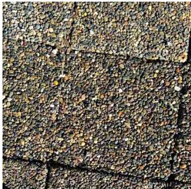
**Figure 10-8 Example of Pervious Paver**
