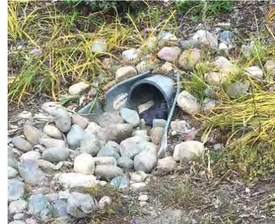
**Figure 8-22** Piped inlet
