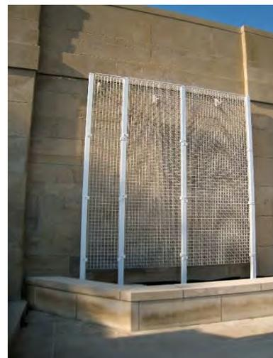
*Figure 12-15 Green façade wall-mounted trellis system*
