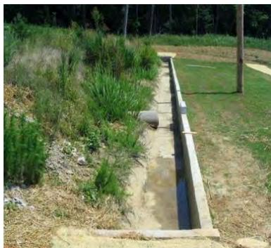
**Figure 9-10 Typical level spreader**
