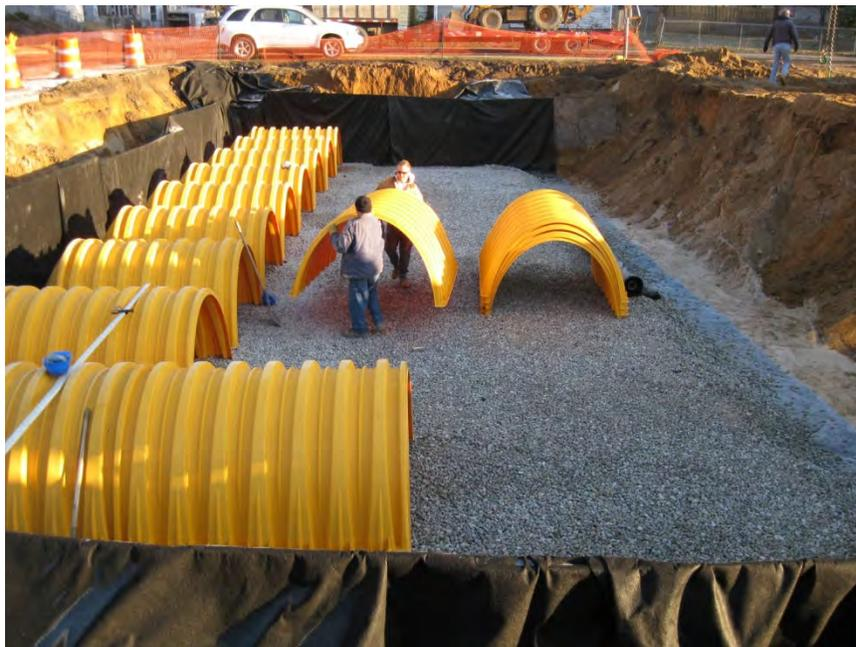
*Figure 7-11 Subsurface Detention During Construction*
