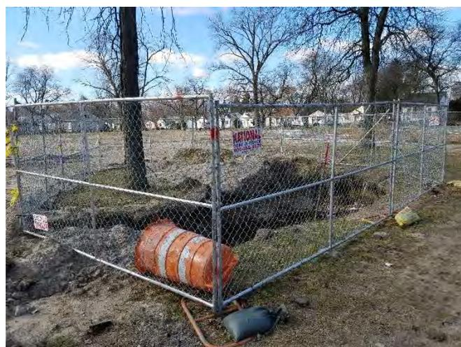
**Figure 15-17 Tree protection removed for excavation**
