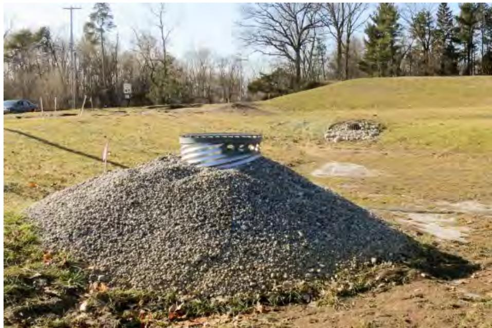
*Figure 7-14 Typical Riser Pipe with Stone Jacket*
