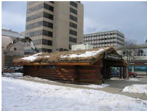
*Figure 12-8 Sloped living roof installation in Alaska*
