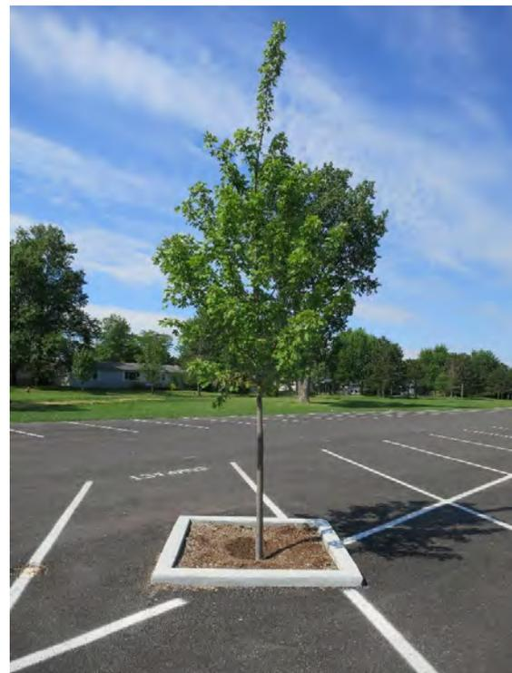
*Figure 8-7 Suspended Pavement Parking Lot*
