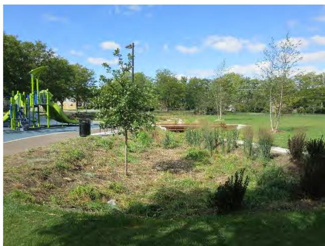
Figure 15-8 Trees in bottom of bioretention
