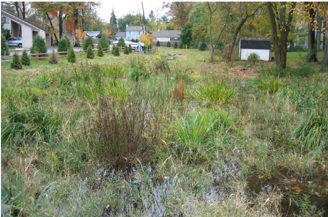
*Figure 13-1 Example Surface Flow Stormwater Wetland*
