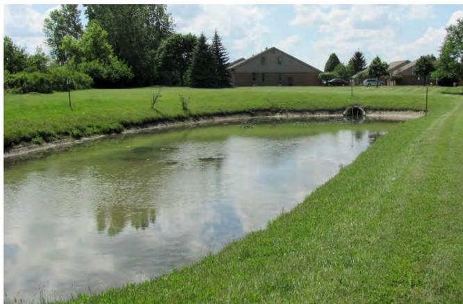
*Figure 7-6 Detention with a Permanent Pool*
