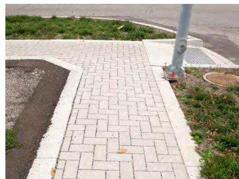
Figure 10-13 Permeable Sidewalk
