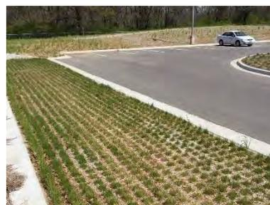
*Figure 10-6 Example of Grid Pavement Systems*
