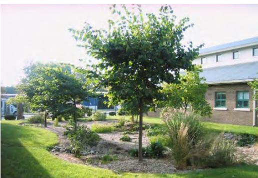
**Figure 8-4 Commercial Bioretention**
