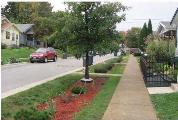
**Figure 8-9 Linear Bioretention Along Roadway**
