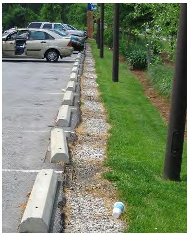
**Figure 8-24** *Vegetated filter strip leading to bioretention*
