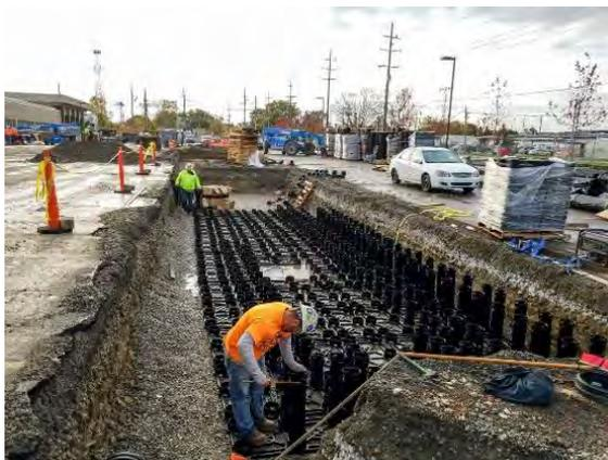
**Figure 15-2** Installation of soil cells
