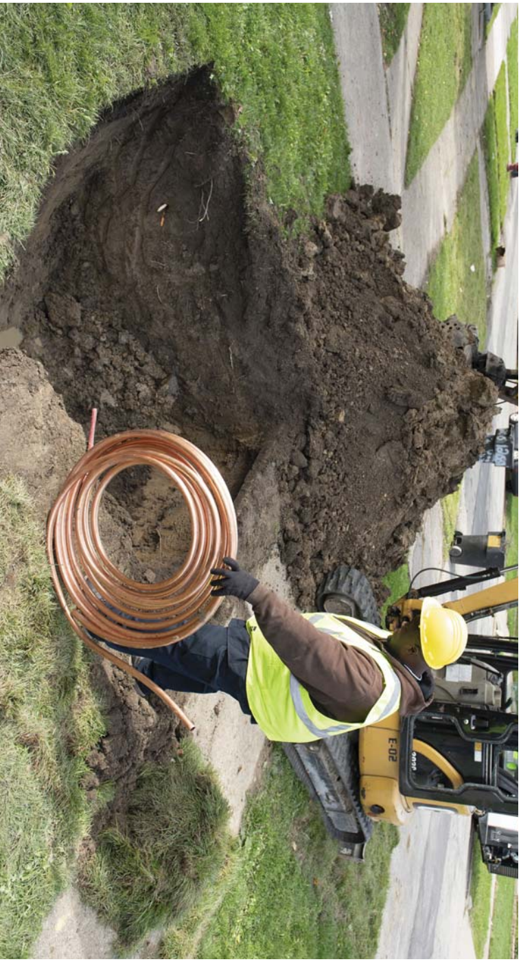
In 2018, DWSD began replacing lead service lines with copper, with owner/occupant permission, while on the same street replacing the water main.
