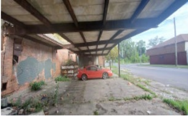
Weight of overhang causing buckling of structure ~ 40 ft high.
