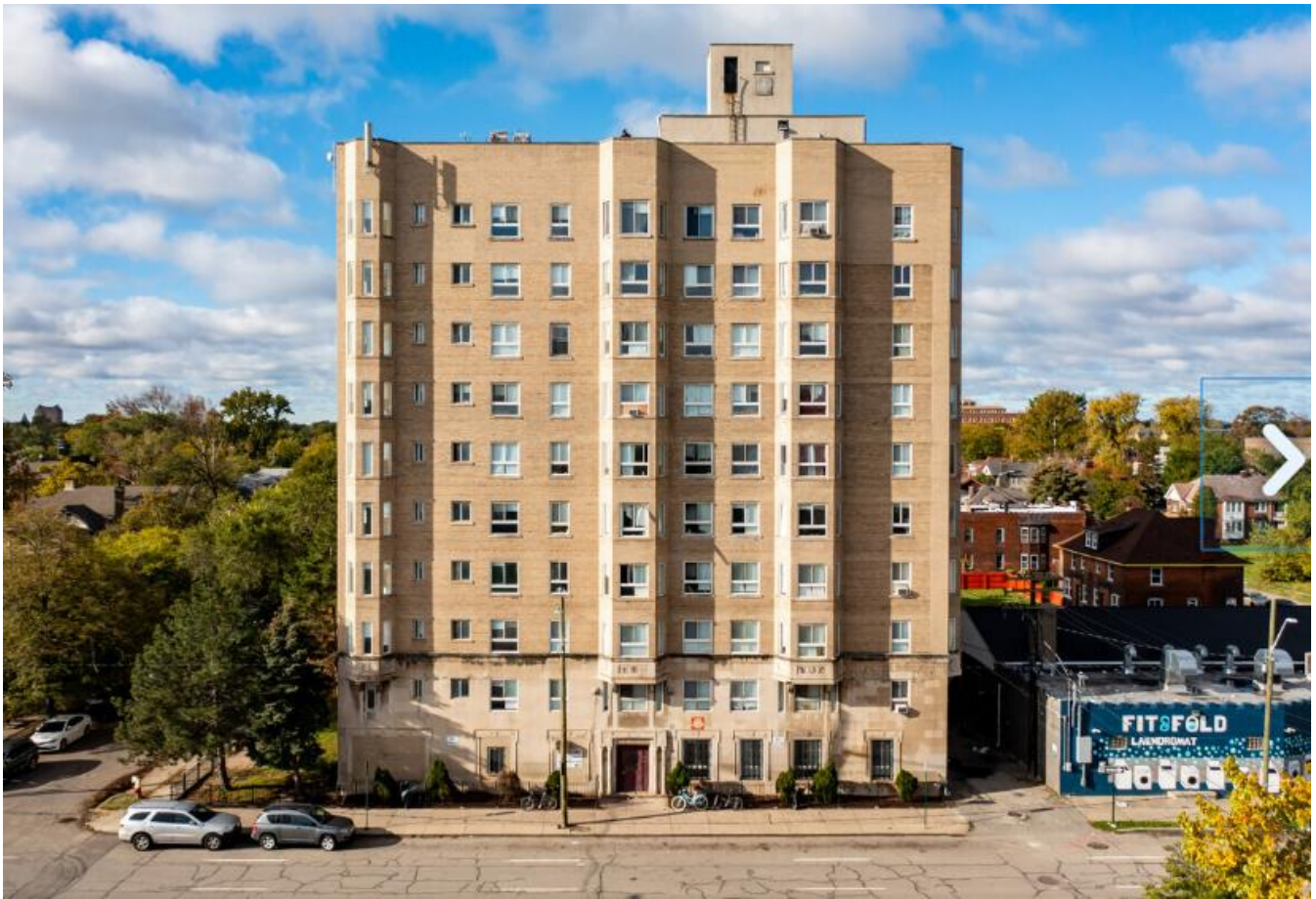
610 Blaine (Lee Crest Apartments) 7
