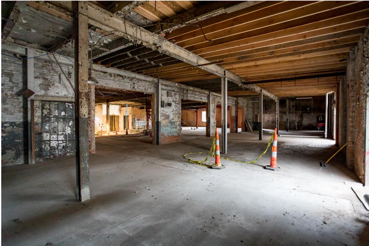
Current interior conditions
