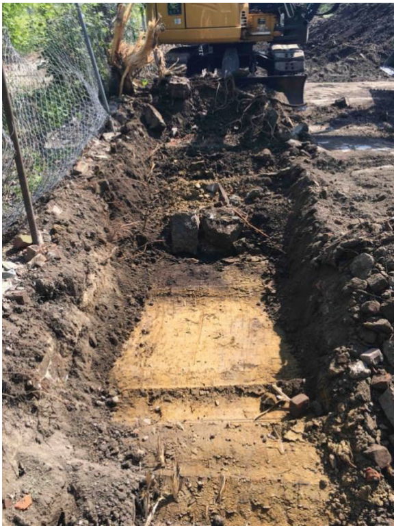
Feature 2 of 20WN1227, facing east toward the stone block footings on the west side of the concrete slab (May 20, 2021).
