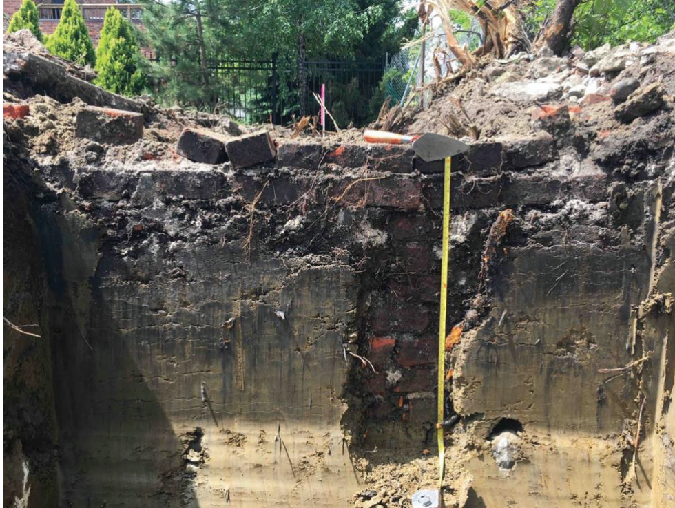
Brick foundation at the northeast corner on the east side of Feature 2, facing west. It extends 9 bricks deep to 85 cm below ground surface and appears to represent its total depth below ground surface given that the top is flush with the concrete slab foundation (May 20, 2021).
