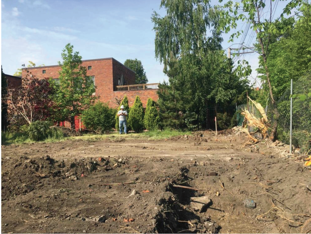
Feature 2, 20WN1227, with the concrete slab foundation is fully exposed. Facing west (May 20, 2021).
