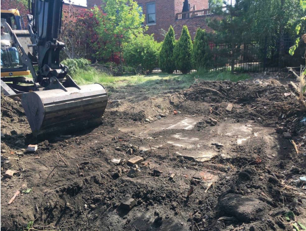
Clearing of the concrete slab foundation of Feature 2 of 20WN1227 (May 19, 2021).
