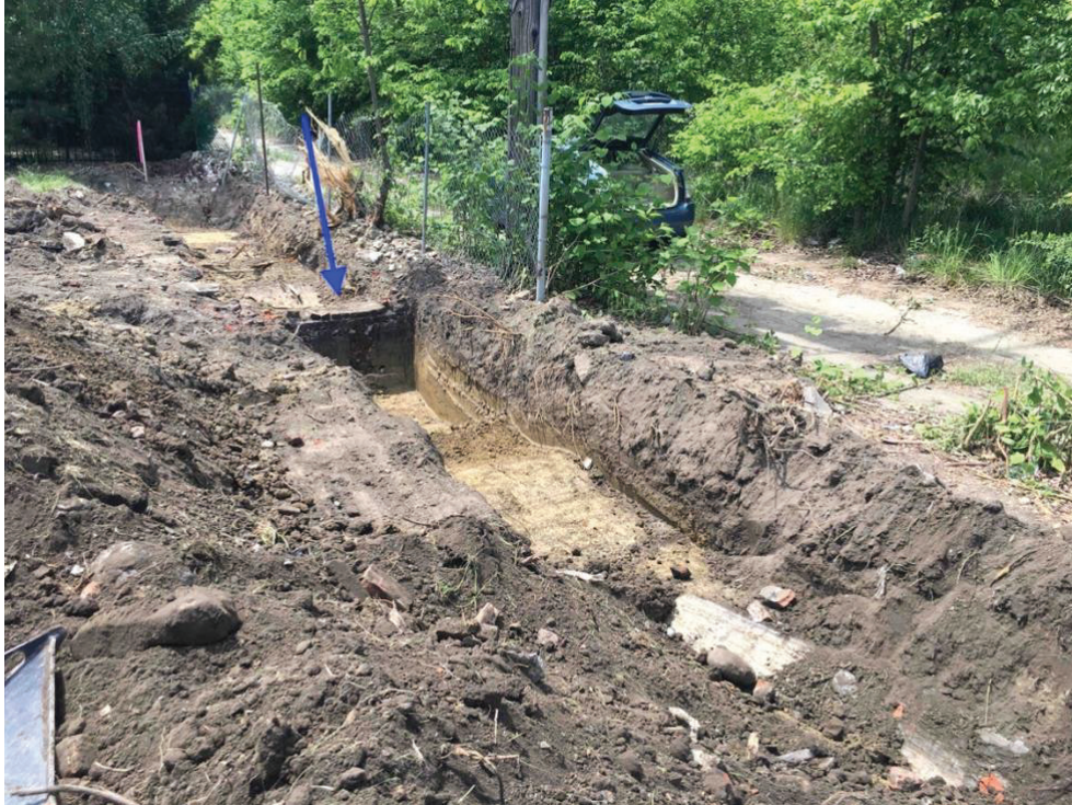
West end of the trench, just west of Feature 1. The arrow indicates the east brick foundation wall for Feature 2 of 20WN1227. Rubble at the east (right) side of the photograph was probably for the footing on the west side of Feature 1. (May 20, 2021).
