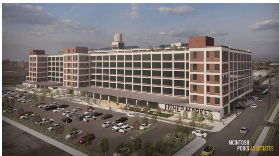
The Fisher Body 21 plant will be reborn as affordable and market-rate housing and destination shopping in the heart of Detroit. It is expected to be completed in 2025. McIntosh Poris Associates
