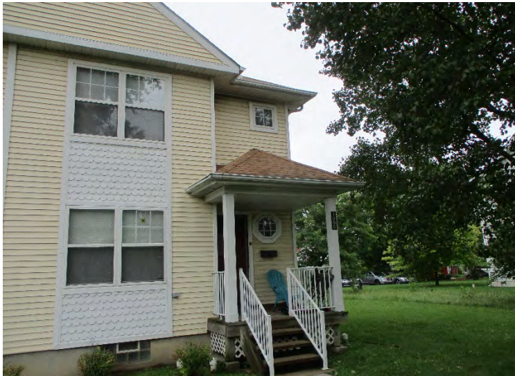
Photo 8. View of 1090-1094 Field Street front
