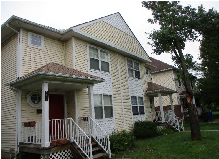
Photo 14. View of 1491-1495 Field Street front
