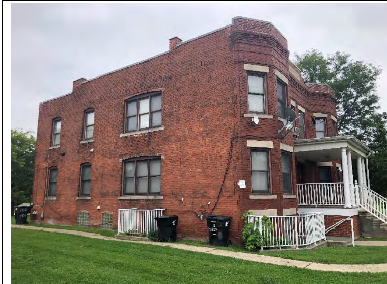
Photo 2. View of 232 East Grand Boulevard, Side B
