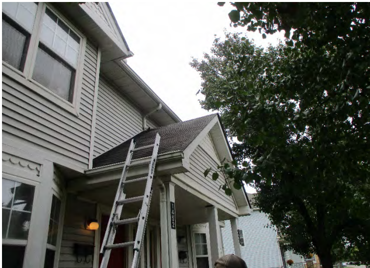
Photo 11. View of 1448-1452 Field Street front
