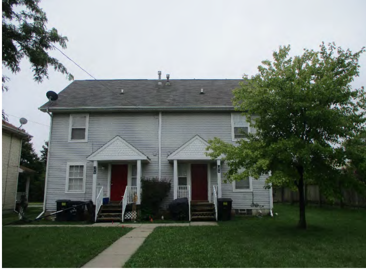
Photo 10. View of 1470-1474 Field Street front
