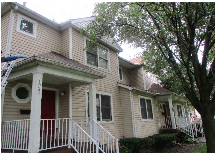
Photo 3. View of 1023-1031 Field Street front
