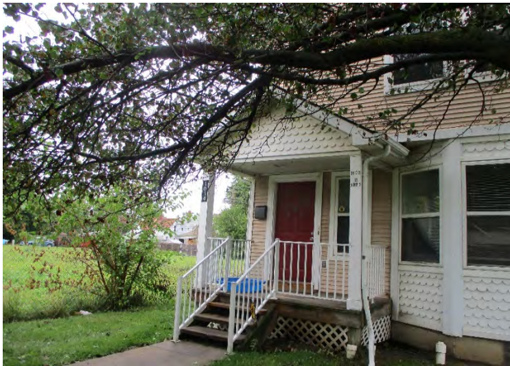
Photo 2. View of 1014-1016 Field Street front
