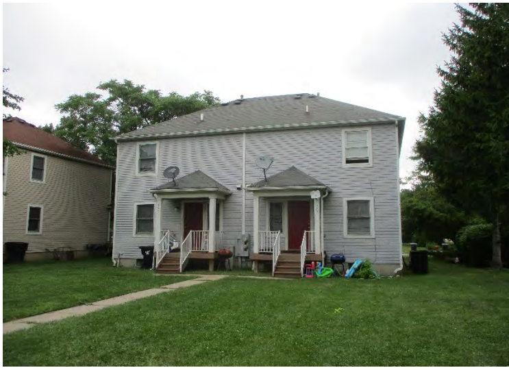
Photo 1. View of 1005-1007 Field Street front
