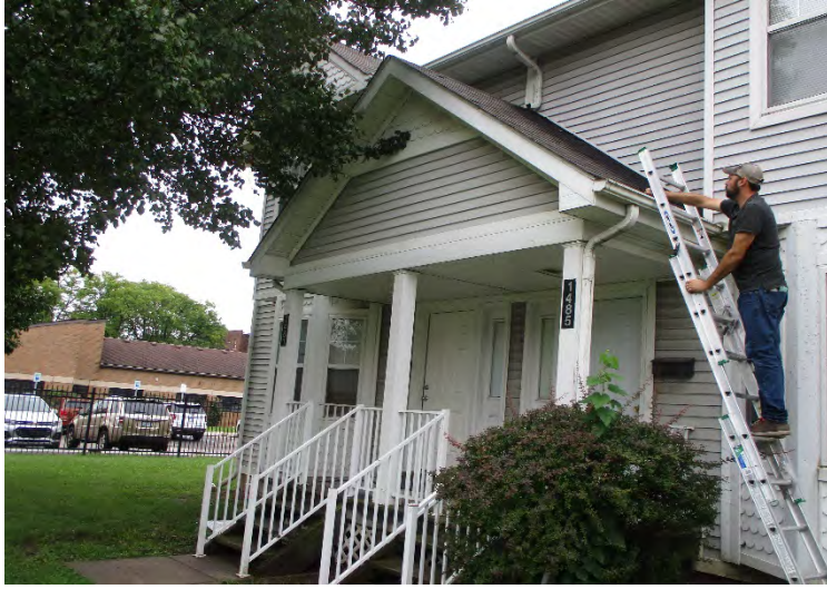
Photo 13. View of 1481-1485 Field Street front
