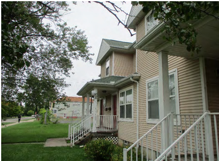
Photo 9. View of 1100-1108 Field Street front
