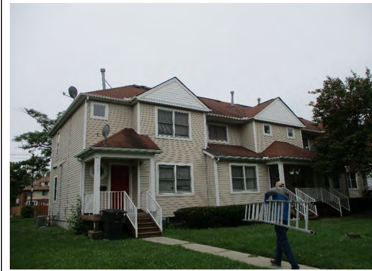
Photo 4. View of 1045-1051 Field Street front
