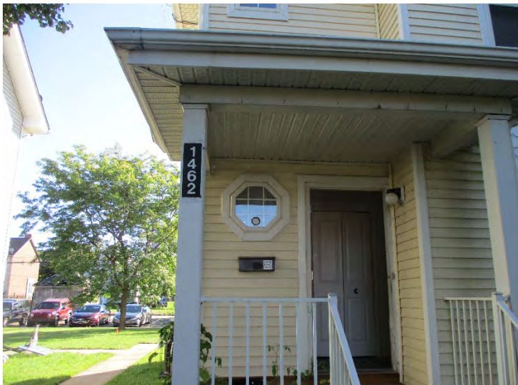
Photo 12. View of 1458-1462 Field Street front
