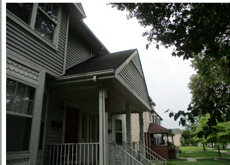
Photo 6. View of 1070-1074 Field Street front
