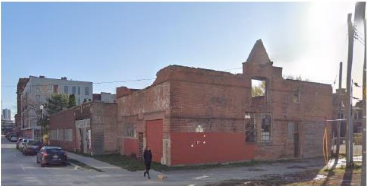
e Existing Carriage House Building (2827 John R. Street)
