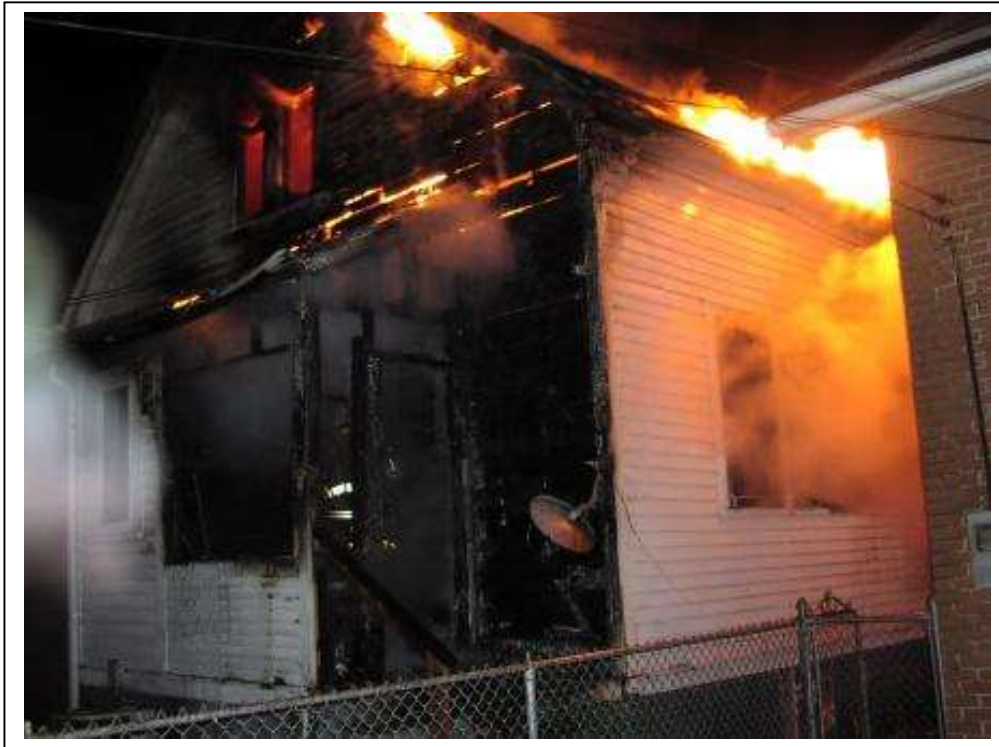
Detroit House Fire, Courtesy of the Detroit Fire Department
