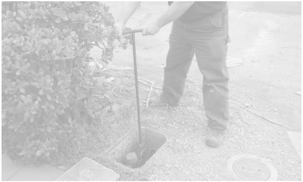
Water theft with unauthorized turn-on
