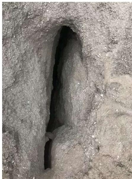
*Exhibit 5 - Surface Cracking around Stockpile*
