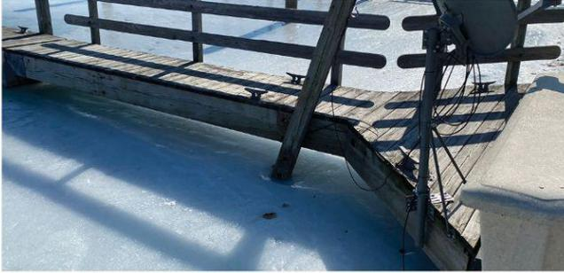
SEVERAL PILES WERE DISPLACED DUE TO ICE SHIFTING
