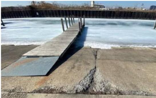
CONCRETE PAD WITH LARGE POTHOLES AT THE BOAT LAUNCH
