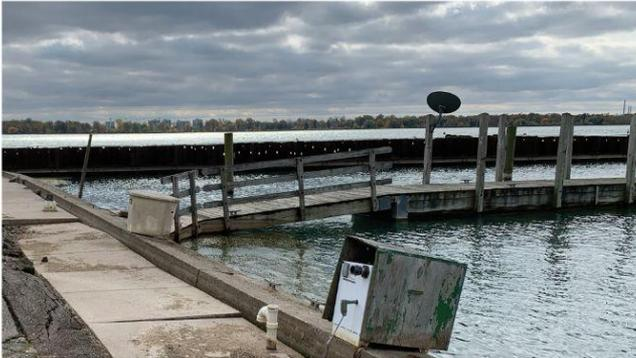
SEVERAL SPUDS AND ANCHOR POINTS WERE OUT OF ALIGNMENT OR IN A LOCKED POSITION
