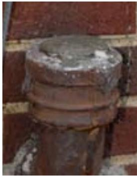
**Straight Pipe:** Cap the sewer pipe. This prevents water from going in. In most cases, you should be able to use a rubber cap secured by a hose clamp. Use a screwdriver or ratchet to tighten the cap until it is secure.
