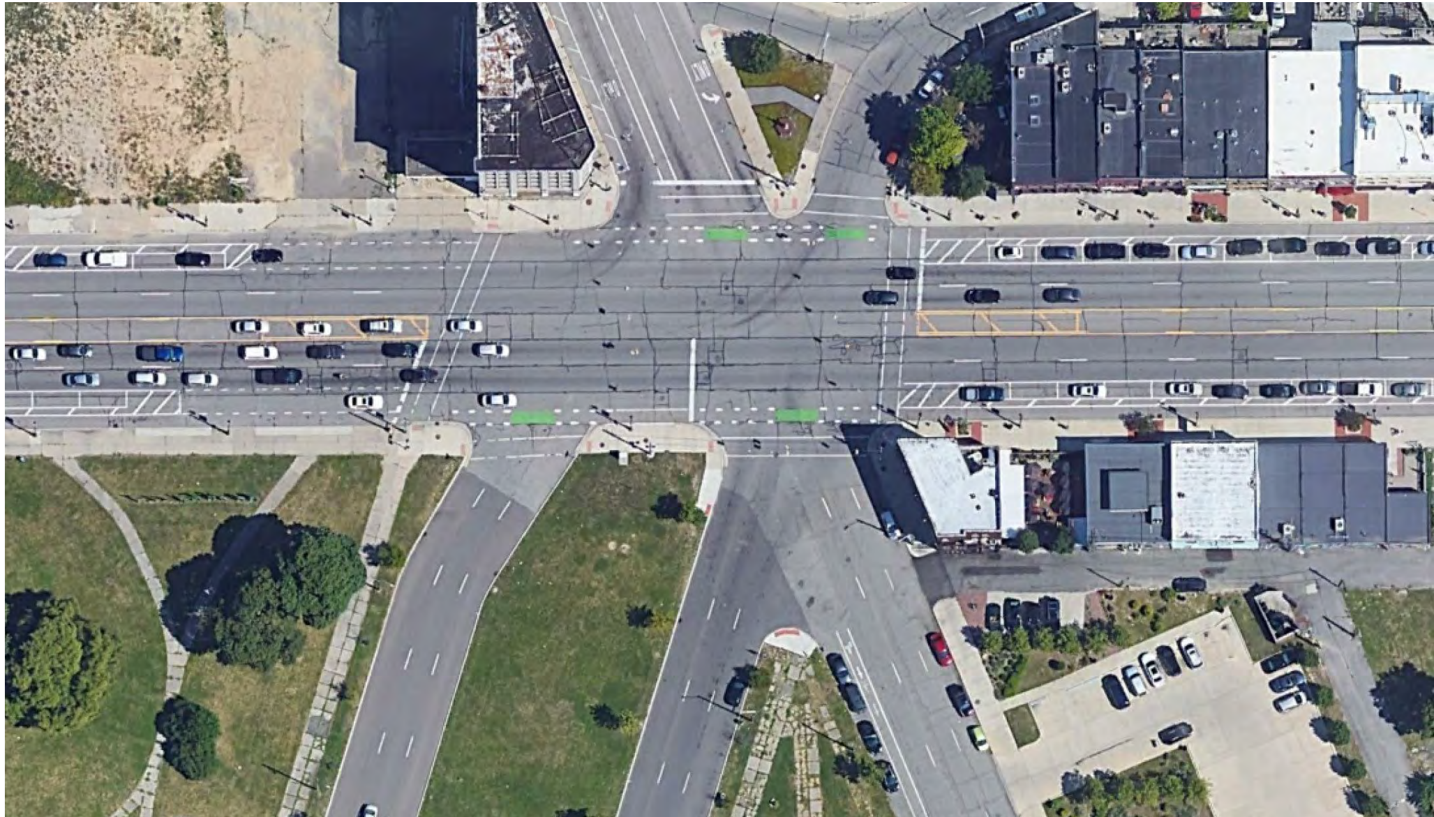
14TH ST AND MICHIGAN AVE - EXISTING
