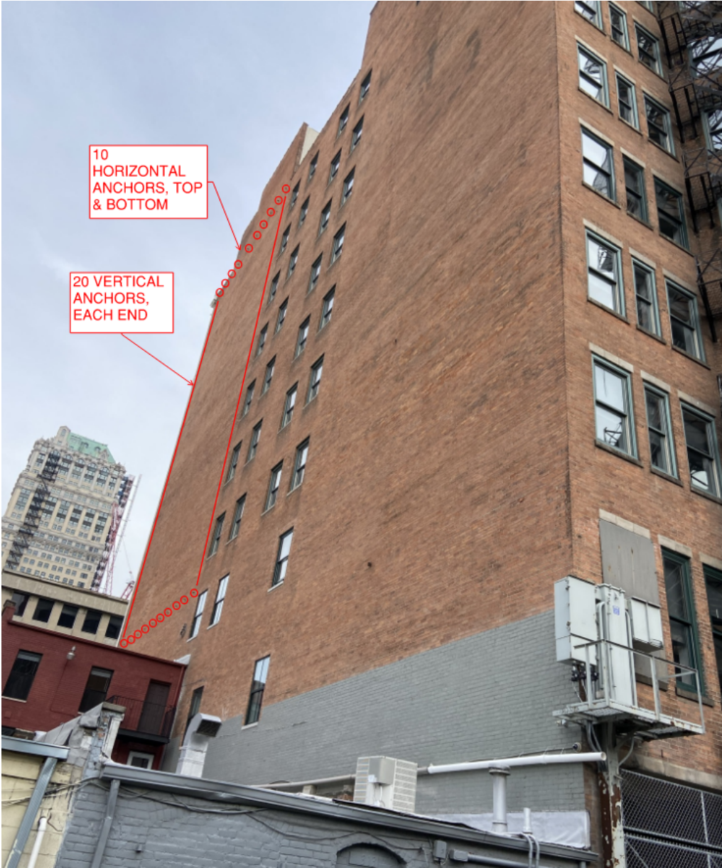
Figure 2 Wall Elevation (Photo by Silman)
