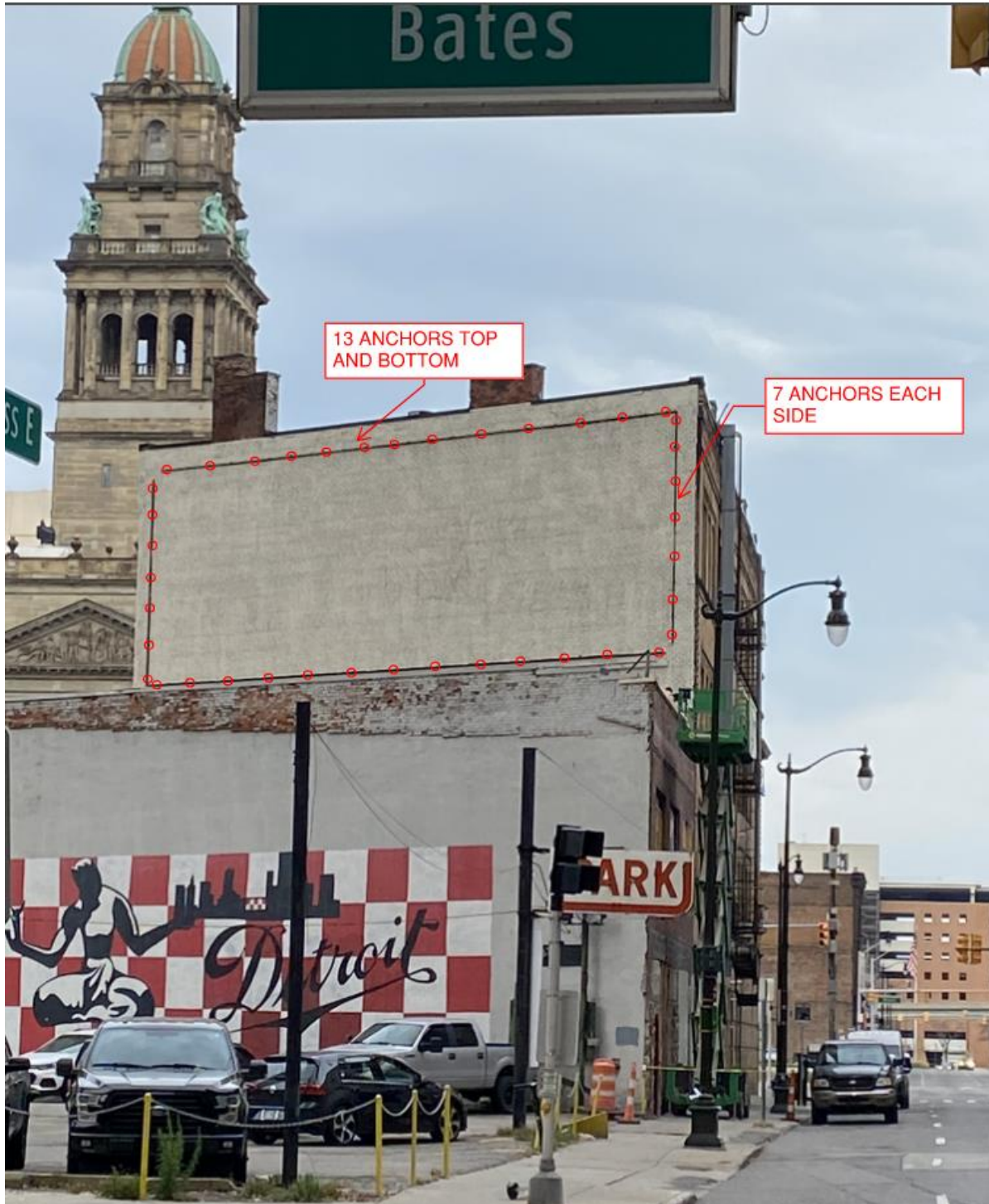
Figure 2 Wall Elevation (Photo by Silman)
