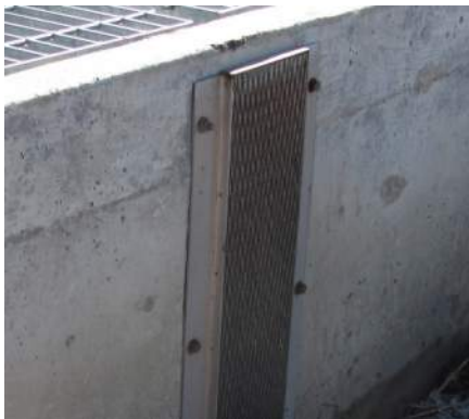
Specialty screen protecting orifice plate from clogging, outside (left); orifice plate, inside (center); clogged poorly designed screen (right)
