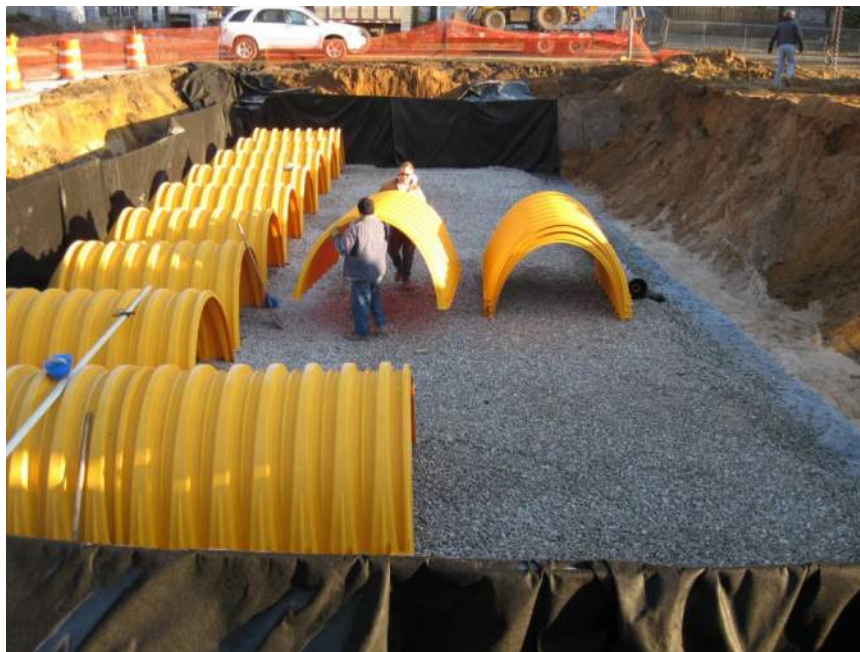
Figure 7-11 Subsurface Detention During Construction
