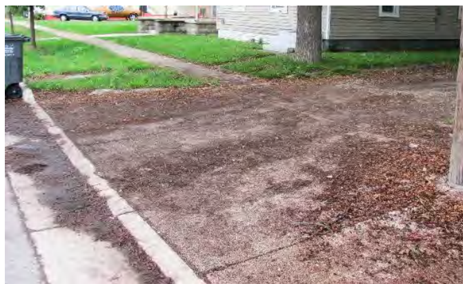
Figure 10-16 Permeable pavement with significant leaf litter
