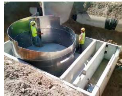
Figure 9-13 Installation of typical manufactured treatment device
