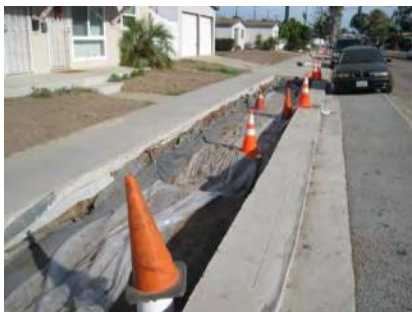
Figure 10-34 Protection of subgrade during construction
