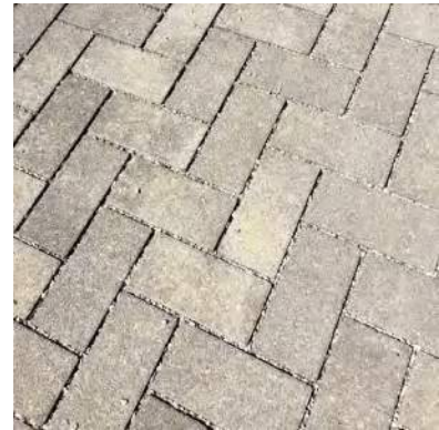
Figure 10-5 Example of Permeable Interlocking Concrete Pavers
