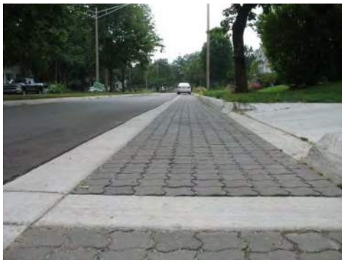
Figure 10-32 Concrete edge restraint between PICP and traditional asphalt
