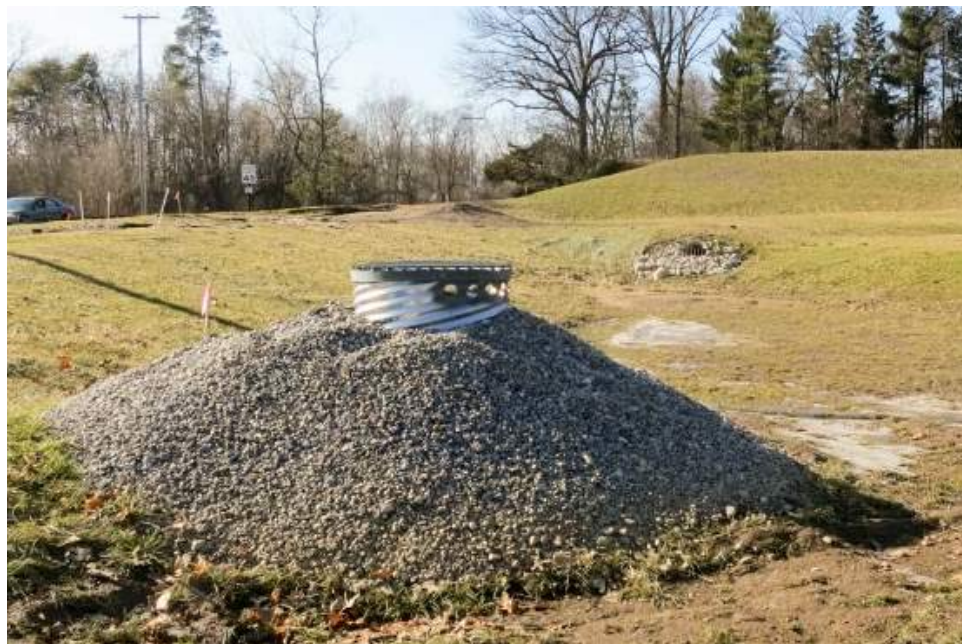
Figure 7-14 Typical Riser Pipe with Stone Jacket
