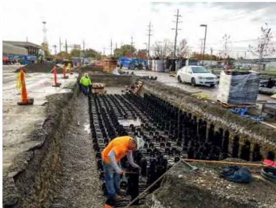
Figure 15-2 Installation of soil cells
