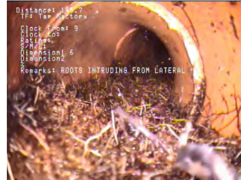
Figure 15-15 Example root growth in sewer
