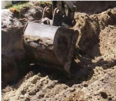
Figure 8-37 Scarifying soil with a toothed excavator bucket
