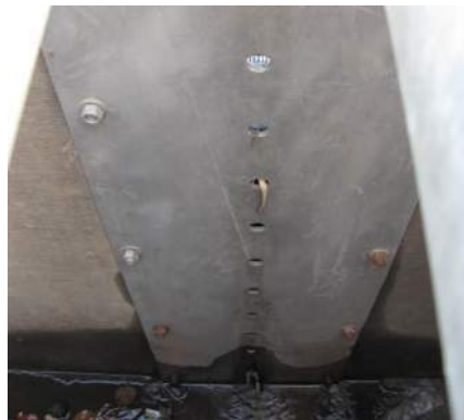
Specialty screen protecting orifice plate from clogging, outside (left); orifice plate, inside (center); clogged poorly designed screen (right)
