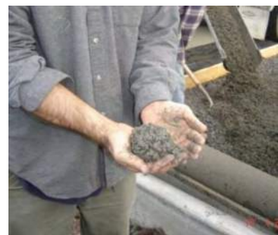
Figure 10-33 Inspection of moisture content in pervious concrete mix during delivery
