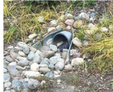
Figure 8-22 Piped inlet
