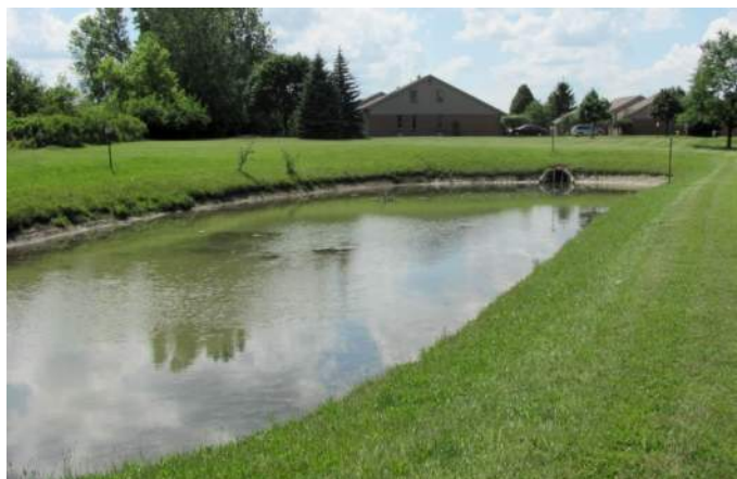
Figure 7-6 Detention with a Permanent Pool
