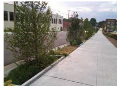
Figure 8-17 Vertical curbing adjacent to sidewalk
