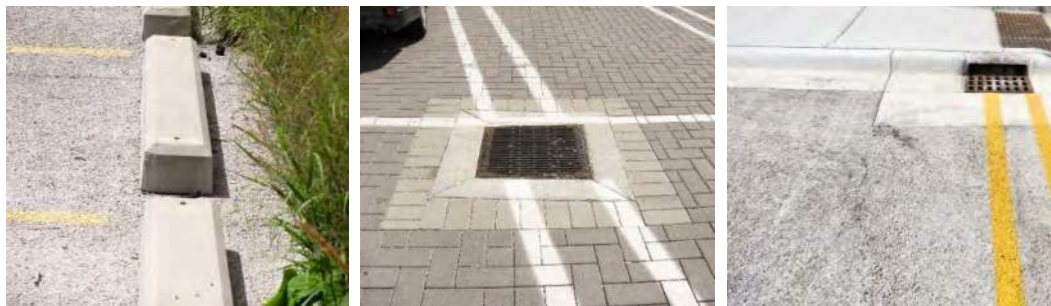
Pervious concrete parking; overflow conveyance to bioretention
