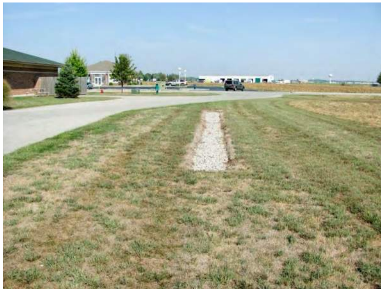
Figure 9-1 Infiltration trench installed adjacent to drive lane
