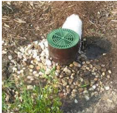
Figure 8-23 Upturned inlet
