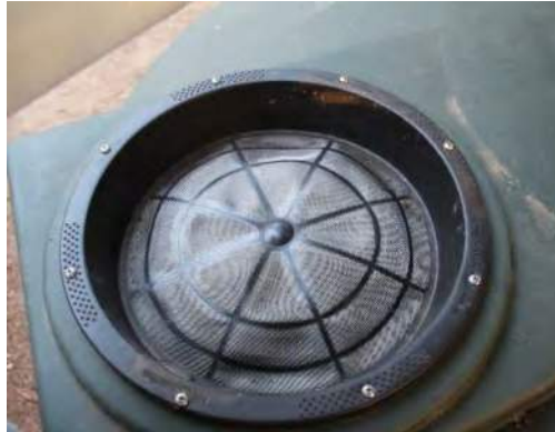
Figure 10-5 Filter at the Inlet on a Cistern
