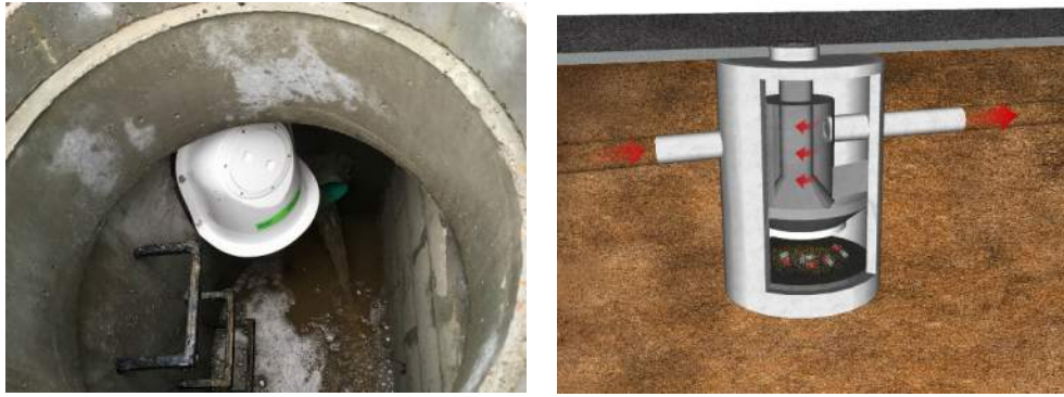
Figure 5-9 Gross Solids Removal Devices
