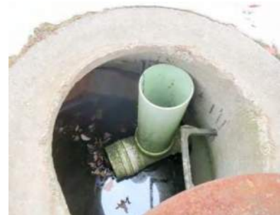
Figure 10-26 Upturned underdrain with a capped tee connection
