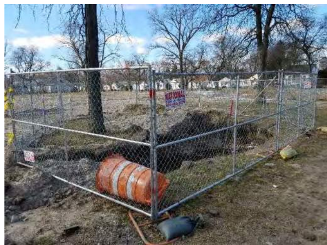
Figure 15-17 Tree protection removed for excavation
