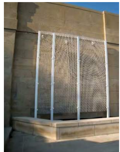
Figure 12-15 Green façade wall-mounted trellis system
