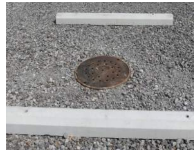
Figure 8-26 Permeable aggregate parking lot outlet structure
