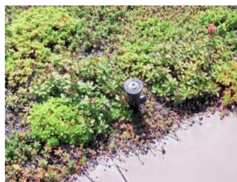
Figure 12-21 Overhead spray irrigation on vegetated roof
