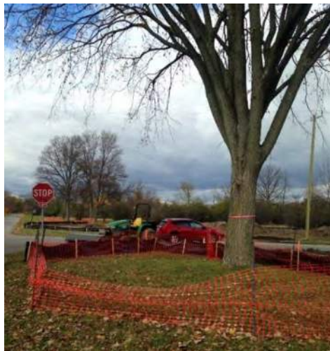
Typical fencing installation, not preferred
