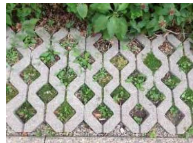
Figure 10-5 Example of Permeable Interlocking Concrete Pavers
