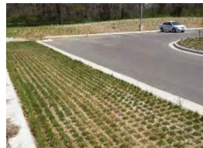
Figure 10-6 Example of Grid Pavement Systems
