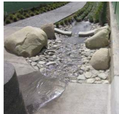
Figure 8-25 Armored inlet
