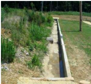
Figure 9-10 Typical level spreader
